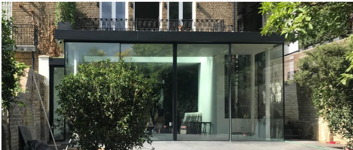
EXAMPLE OF SLIM LINE ALUMINIUM GLAZING SYSTEM
