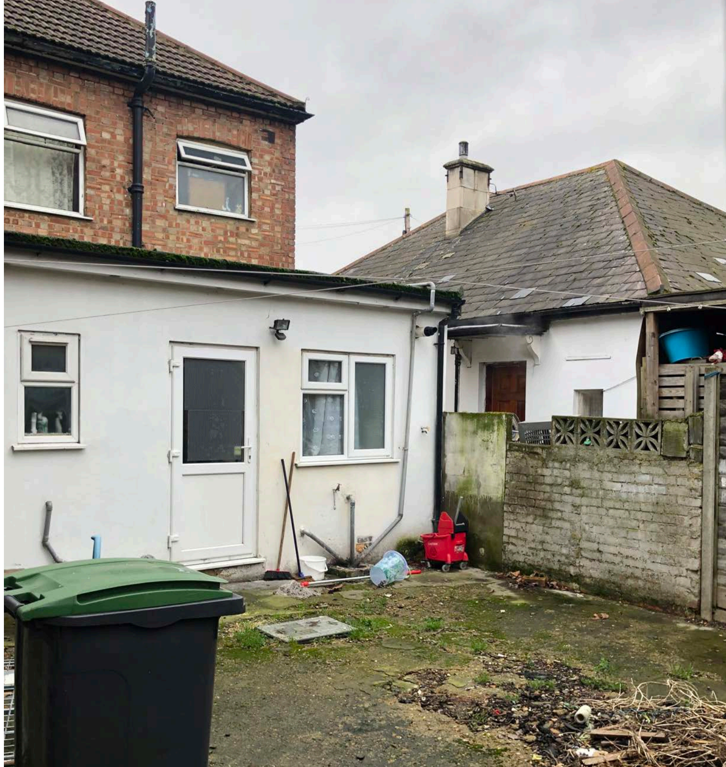
No.7 seen from the rear yard of No.9 Brantwood Road
