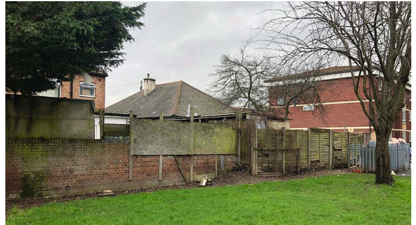
Rear of No.7 and No.9 Brantwood Road
