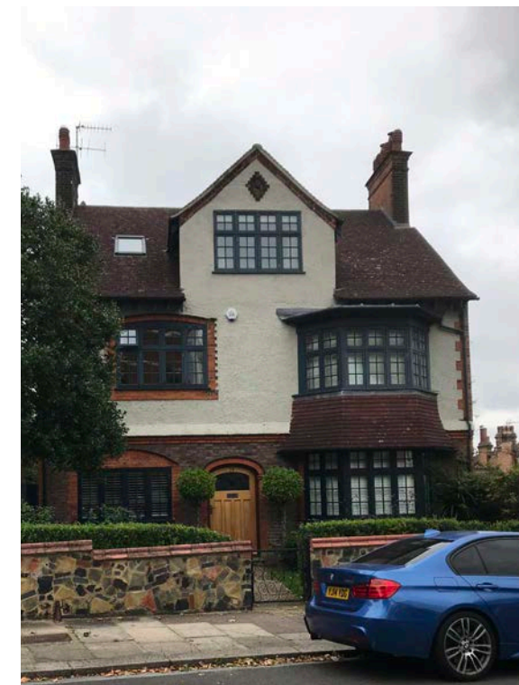
Unusal Arts and Craft elevation and roof treatment in local area
