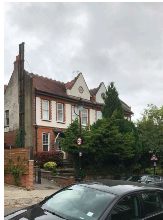
Assymetry and Symmetry in Arts and Craft elevation and roof treatment in Cholmeley Cresc
