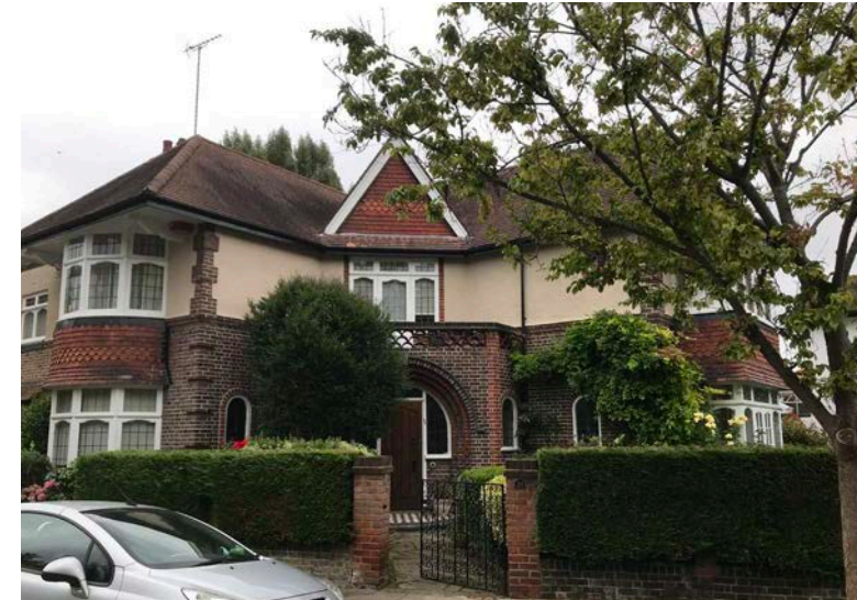
Complex mannering of the elevation on the Corner of Cholmeley Crescent and Cholmeley Park
