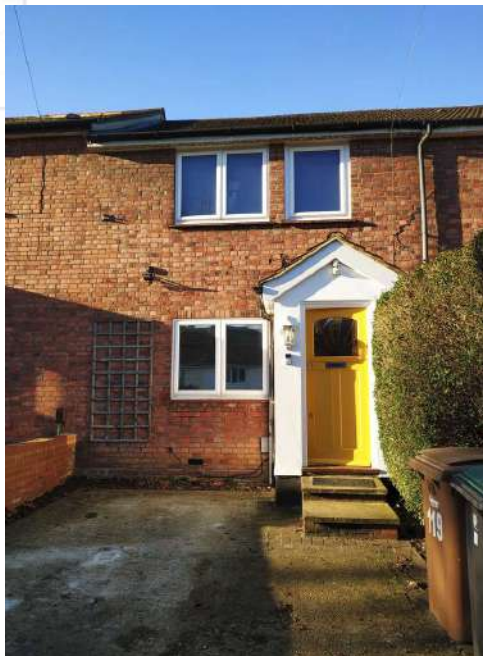
Figure 5 - view of front elevation
