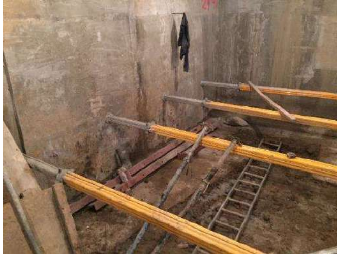
Figure 26: Example of propping (relevant to main basement)
