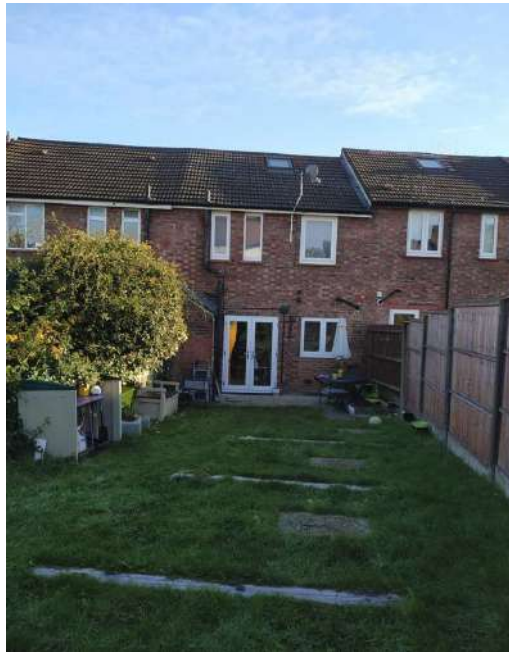
Figure 6 - view of rear elevation
