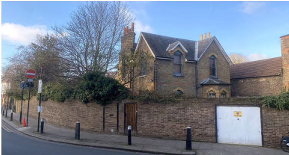
Photo 4 - looking towards north-east / south-east elevations from Moorefield Road
