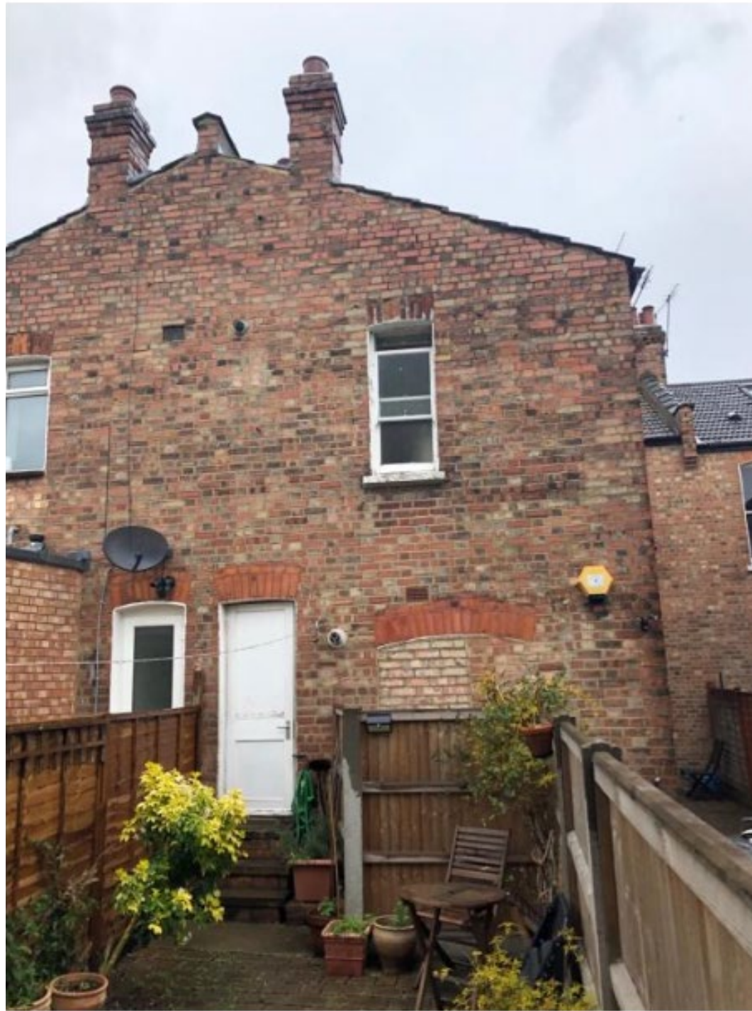
View of the rear façade of 61 Albert Road
