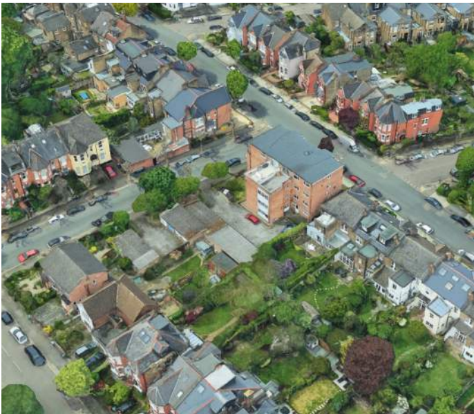
Site Photo 4 East Aerial
