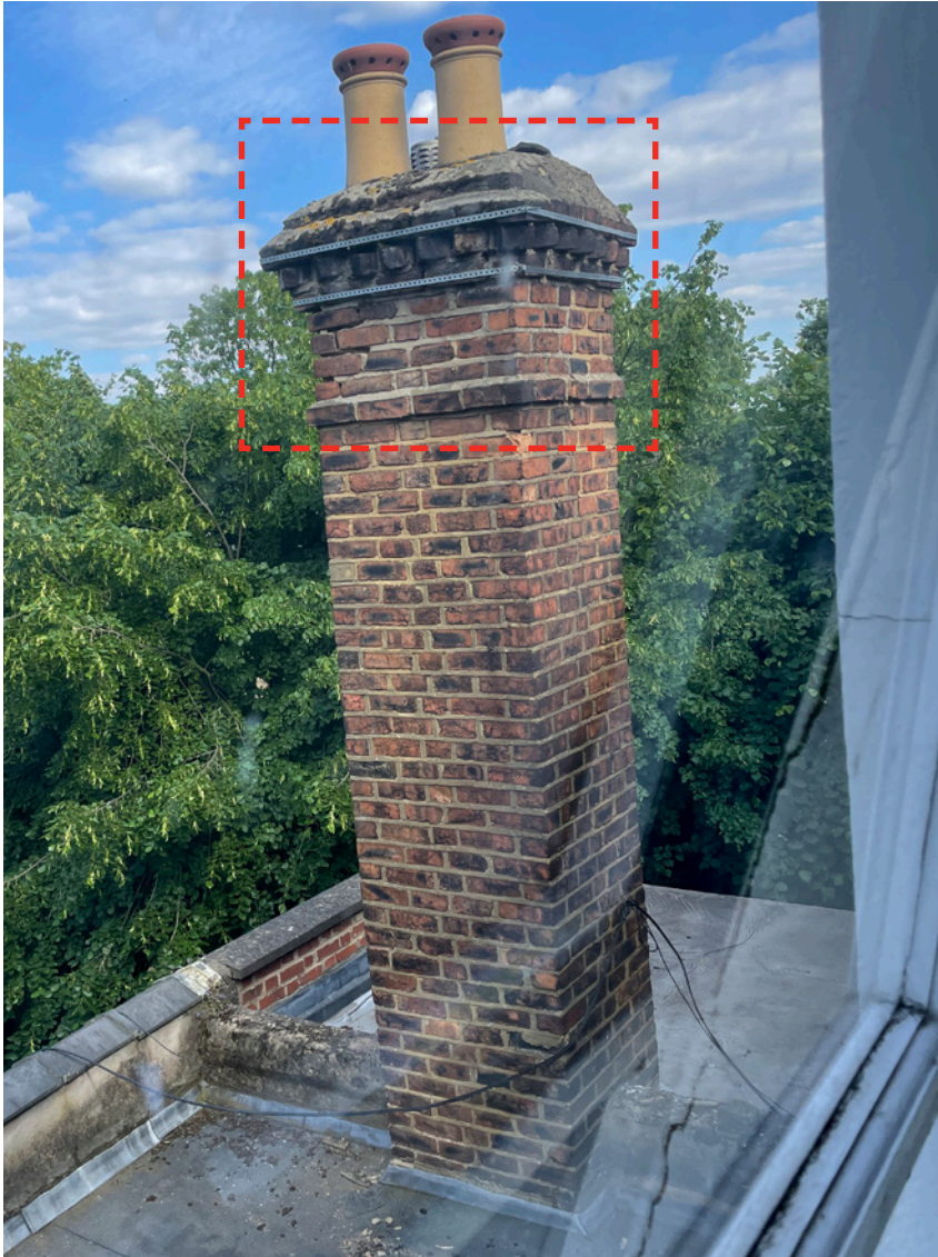
Fig 13 : Picture of existing chimney stack between No. 2 and No. 4 Mount Pleasant Villas
