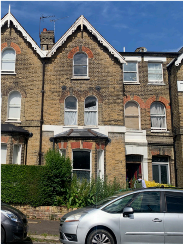
Fig 5 : Existing front facade showing the architectural expression of the terrace and the neighbouring properties
