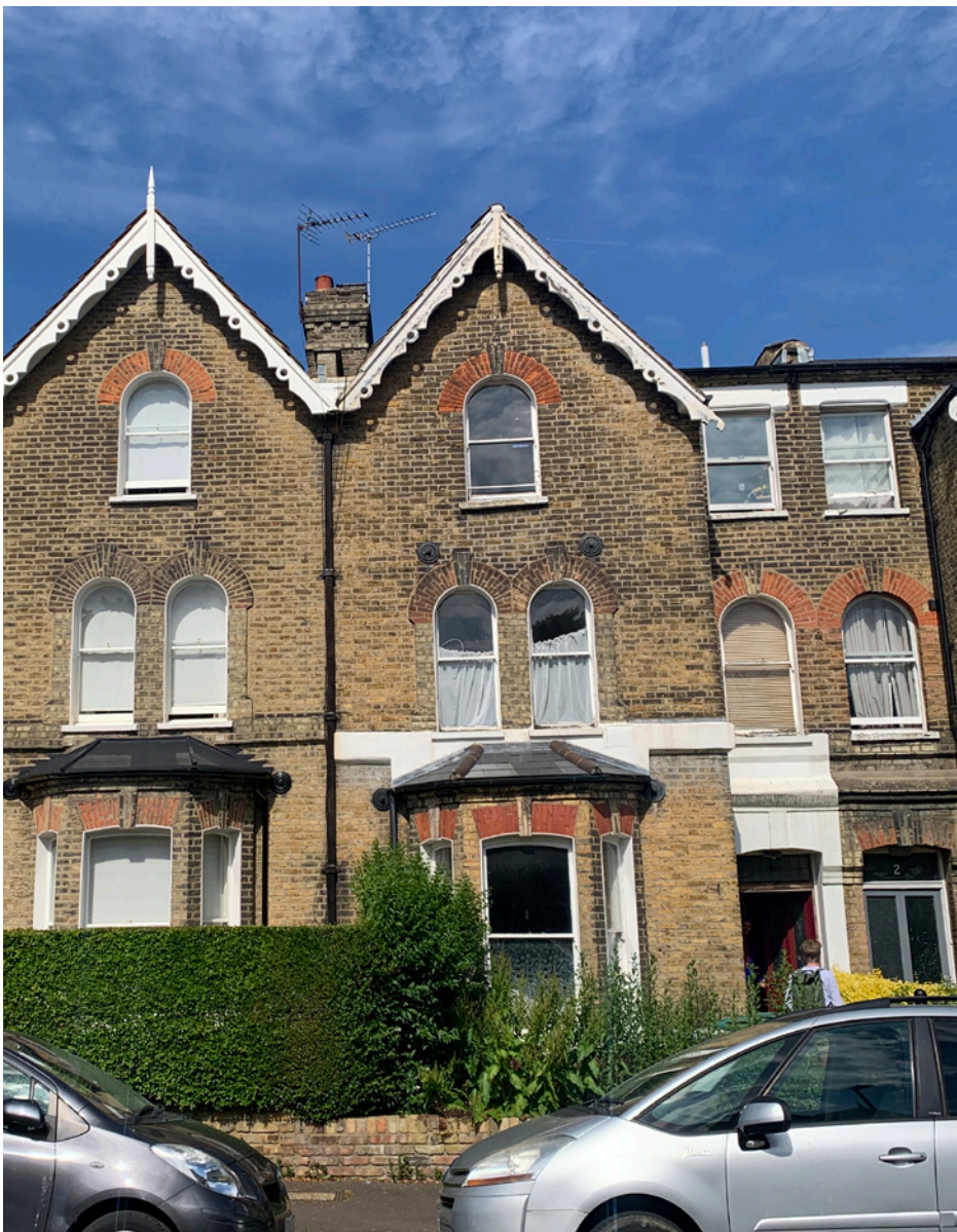
Fig 1 : View from the street towards no 4 Mount Pleasant Villas
