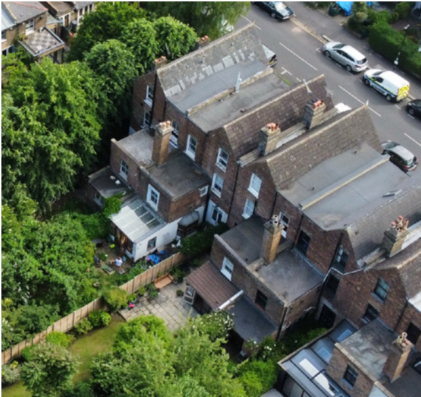
Fig 7 : Aerial photo to the rear of the application site.
