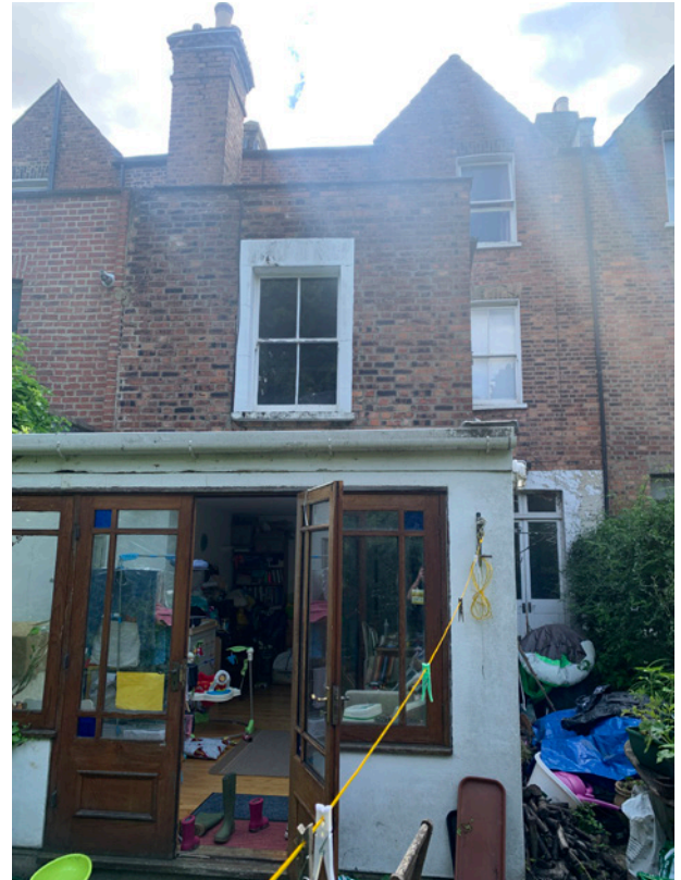
Fig 6 : Existing rear facade with lean-to extension and side access from the kitchen.
