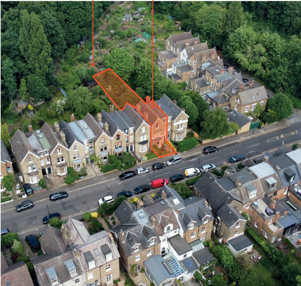
Fig 2 : View from the street towards no 4 Mount Pleasant Villas
