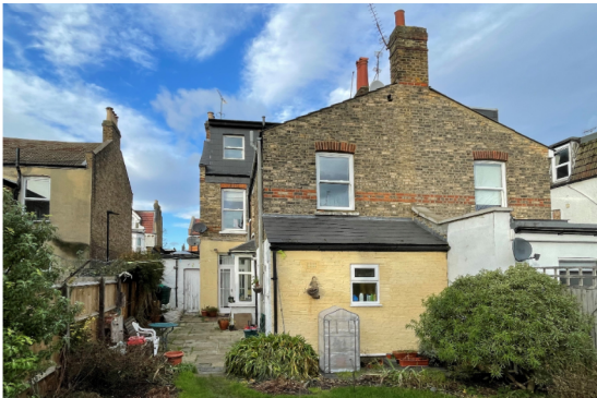
View 2 Looking towards the house
