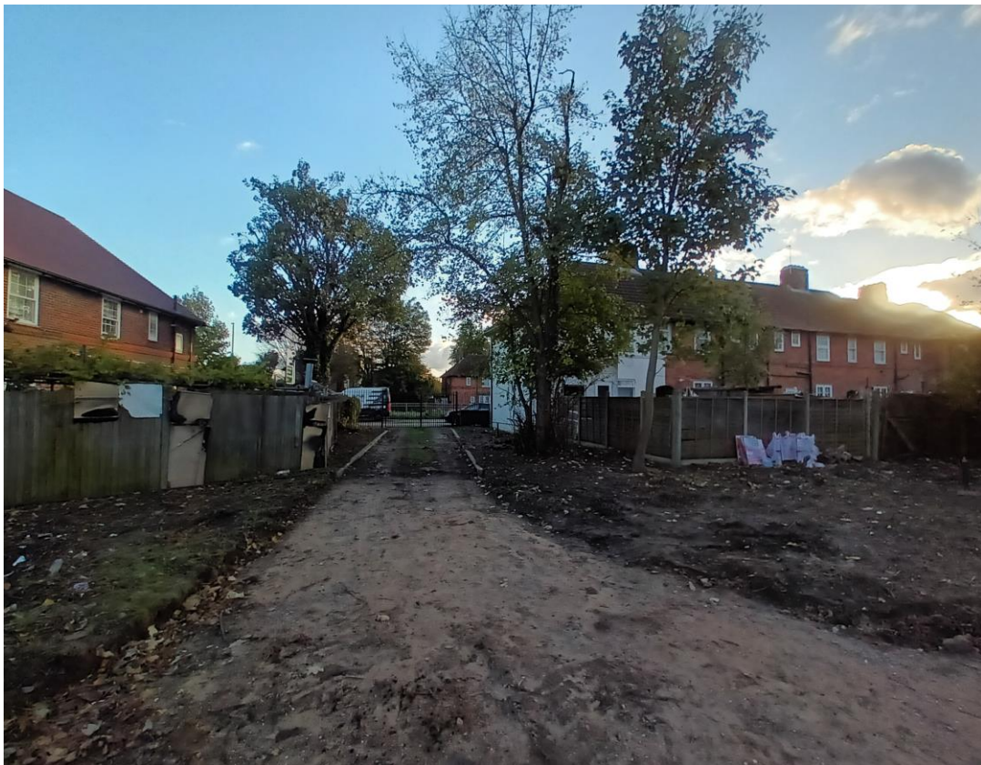
Showing site entrance and adjacent plots
