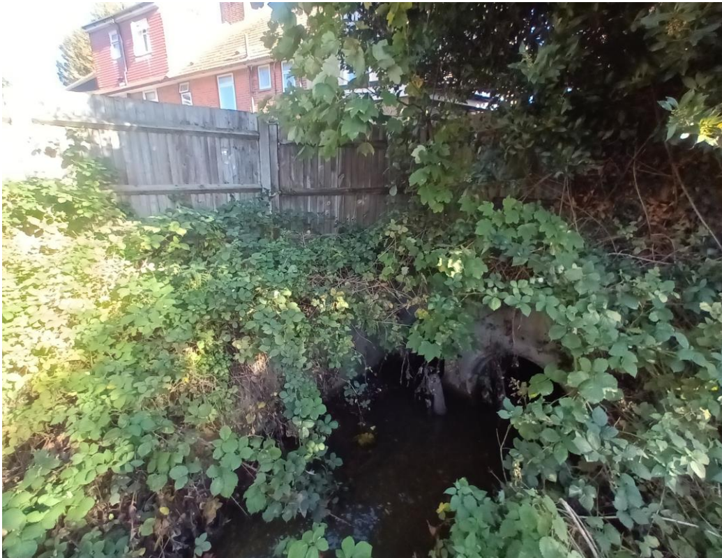
Showing culvert on the northeast site boundary
