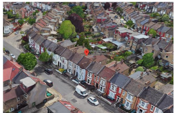
6. Front Aerial View of Site at Gloucester Road
