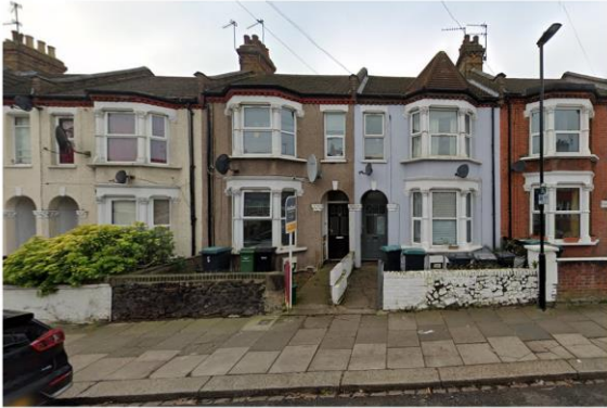
1. Front View of Site at Kings Road
