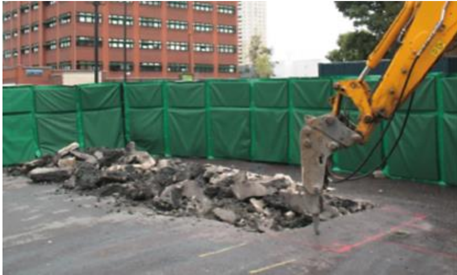
Example Photo of Noise screens erected
