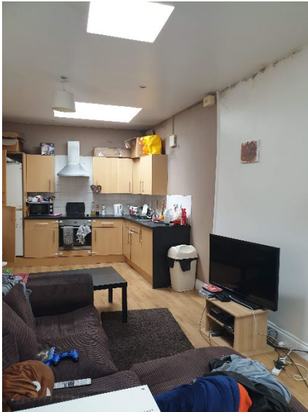
Existing Living/Kitchen and dining space- First Floor
