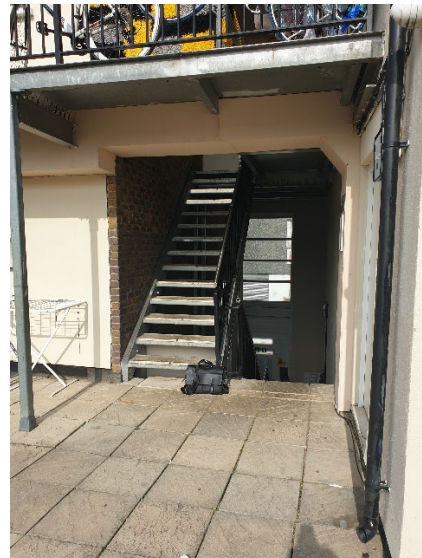
Existing access to the property
