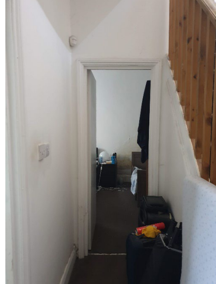
Existing Corridor – Ground Floor
