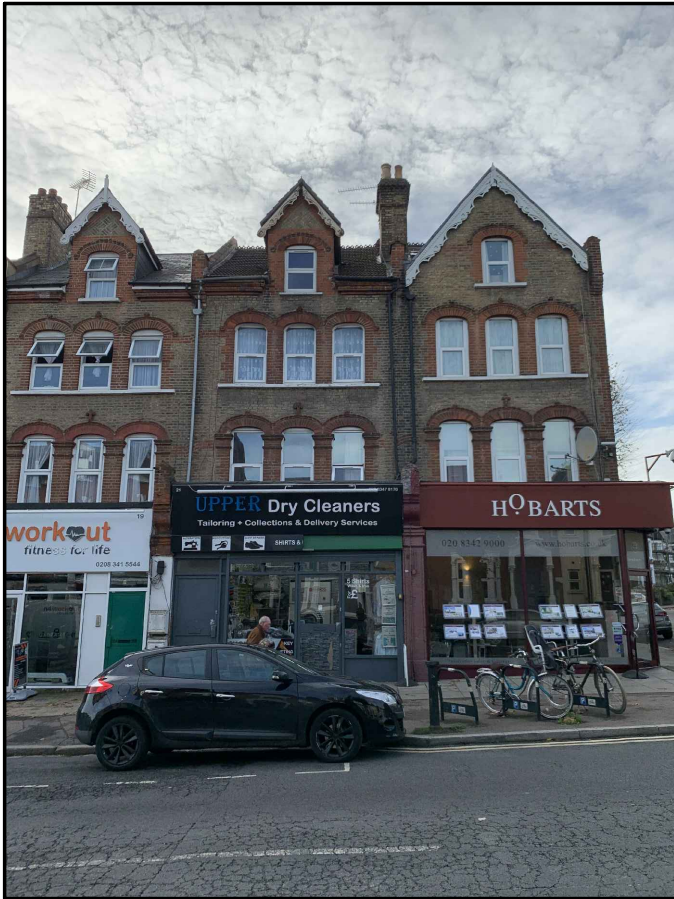
EXISTING SITE PHOTO
