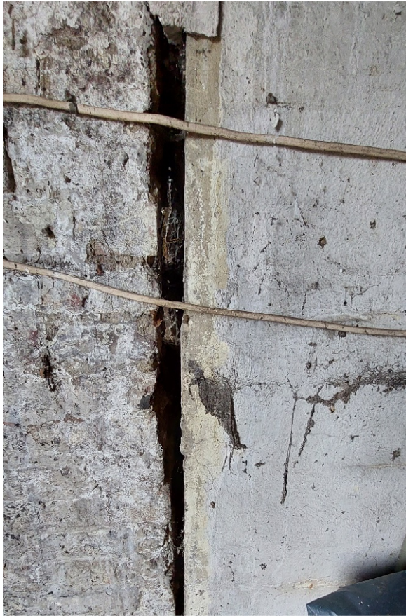
Gap between nib-wall and wall of the Asset
