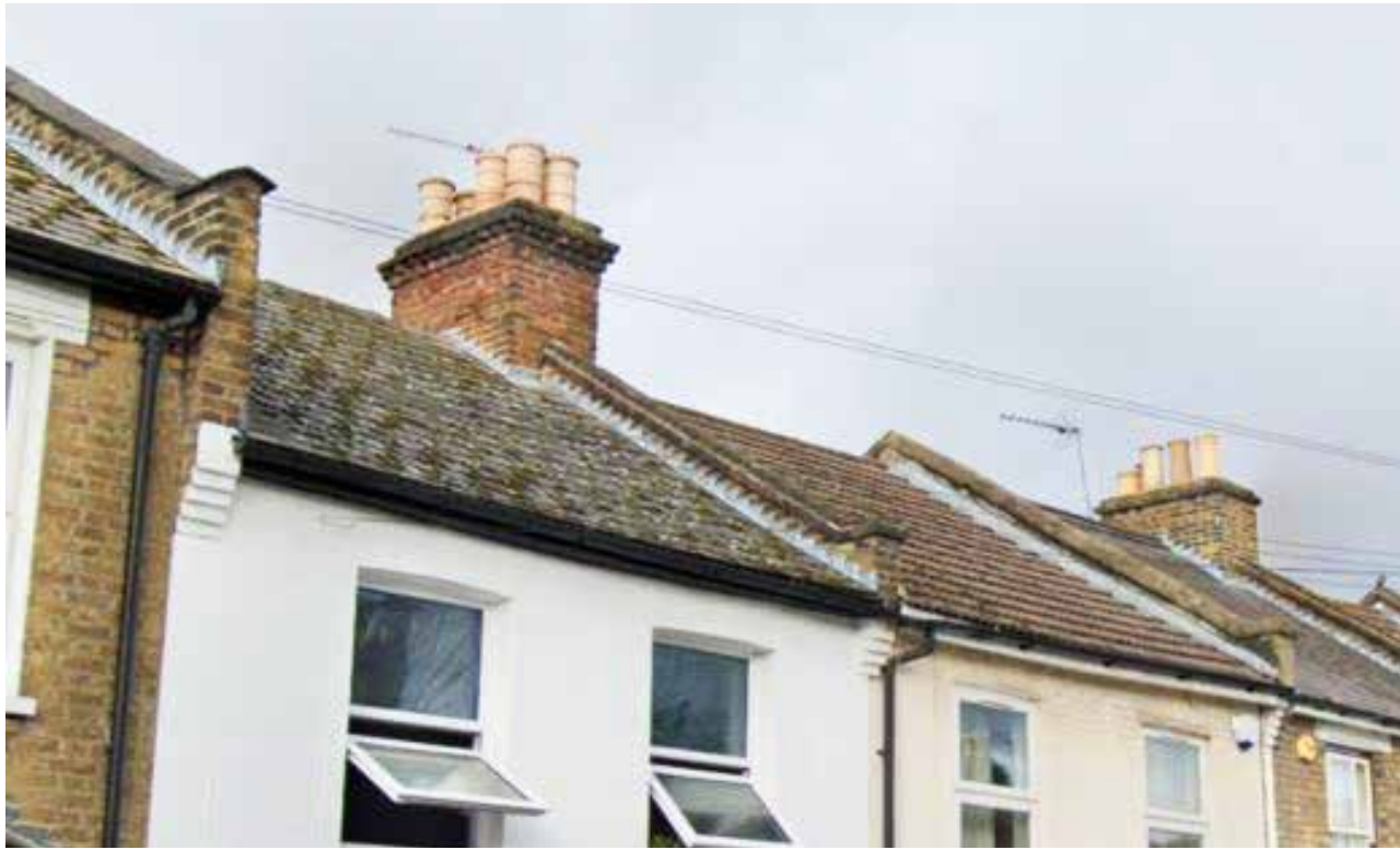
SLATES AND TILE ROOF
