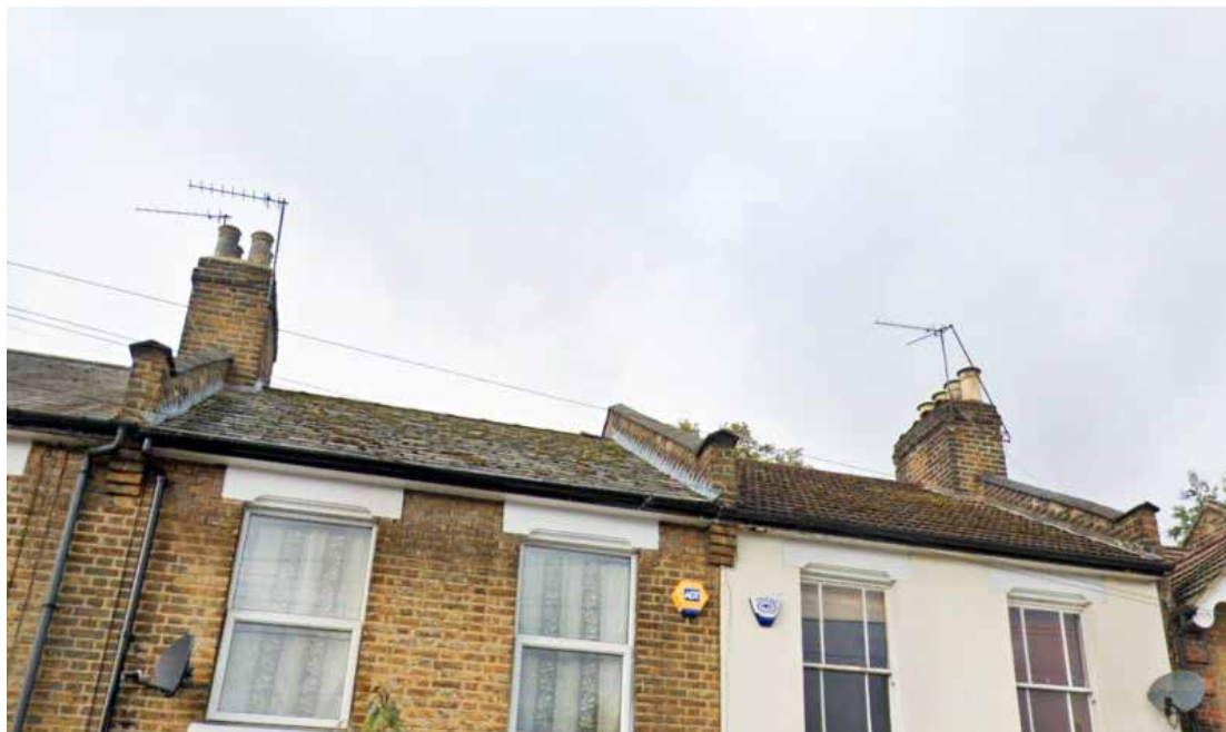
SLATE AND TILE ROOF
