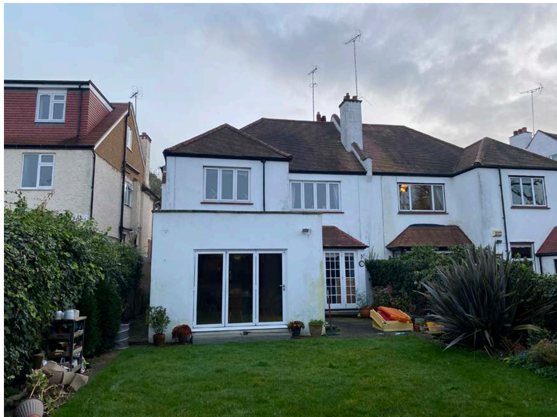
Existing rear elevation of 74 Vallance Road
