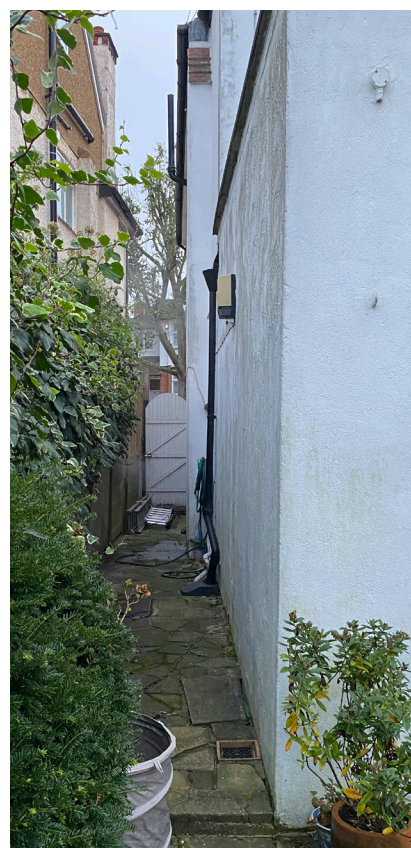
View down side access passage
