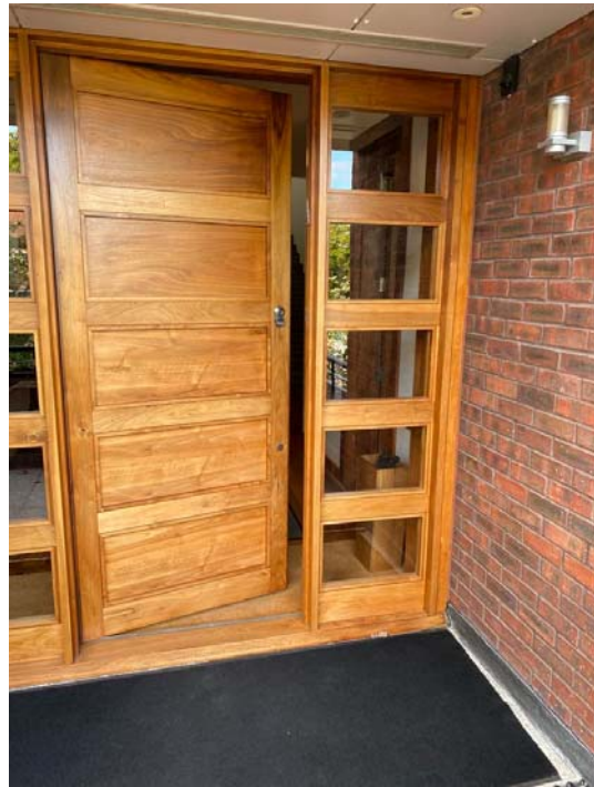
Entrance door in stained natural timber.
