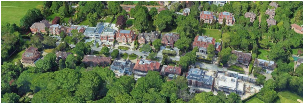
Aerial view of Courtenay Avenue looking west
