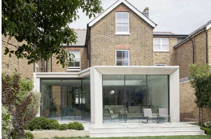
1. Rear extension showing precast stone surround
