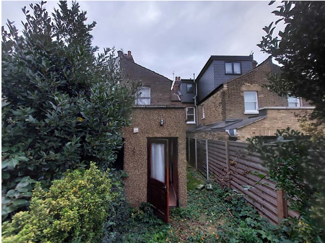
View showing existing extension in the garden
