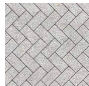
Herringbone paving to communal path
