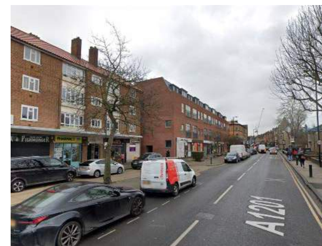
3 The existing newer development makes up a key part of the Park Road high-street
