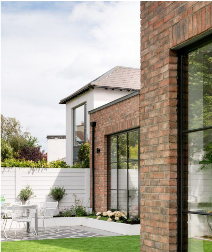
2. Crittall style openings in red brick extension
