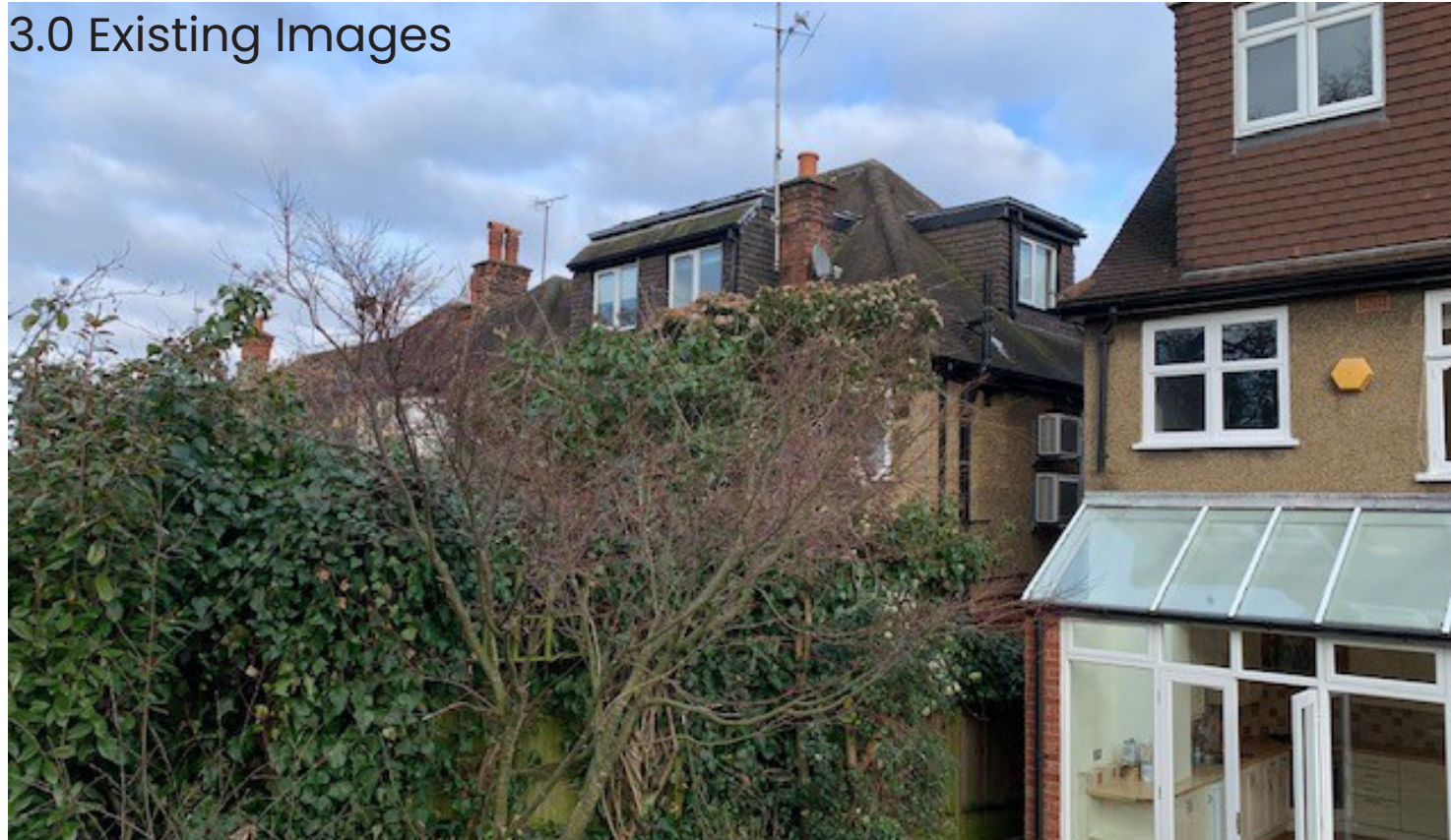
1. Existing rear elevation looking left to No.33 Ringwood Avenue
