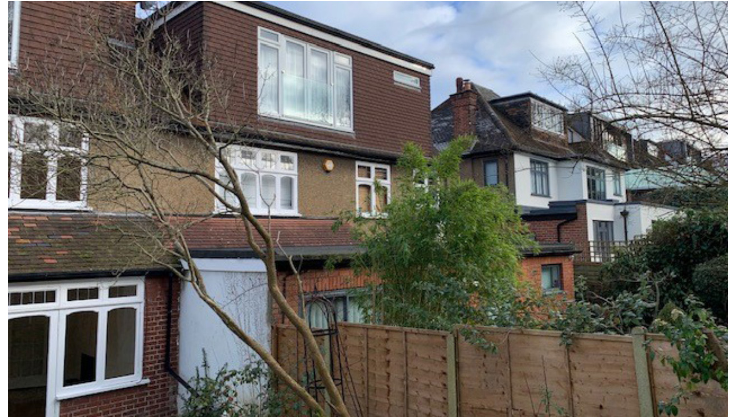
2. Existing rear elevation looking left to No.29 Ringwood Avenue
