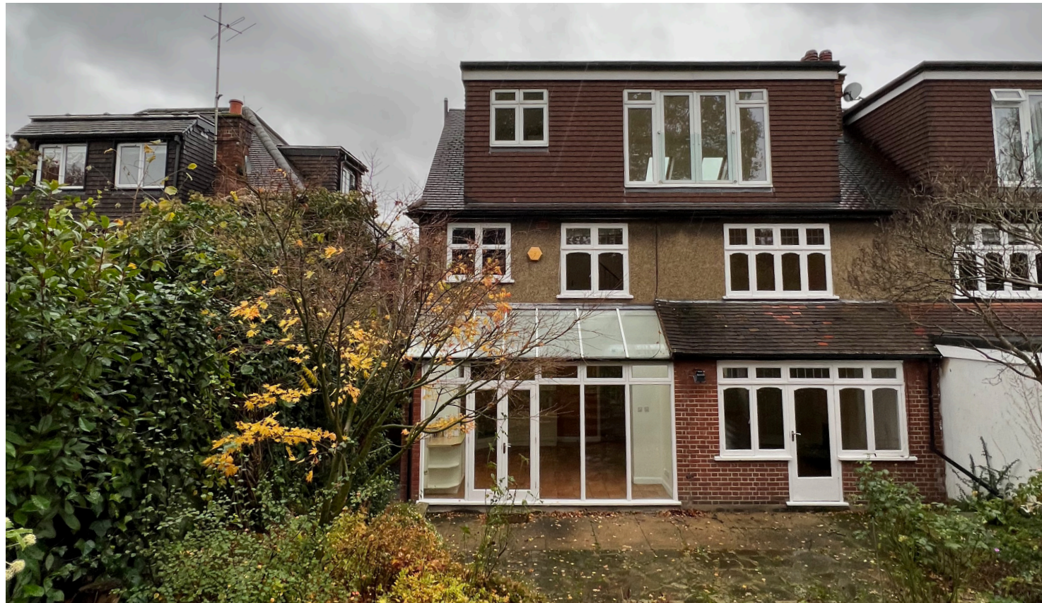
3. Rear elevation of No.31 Ringwood Avenue
