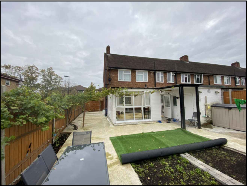
EXISTING REAR VIEW
