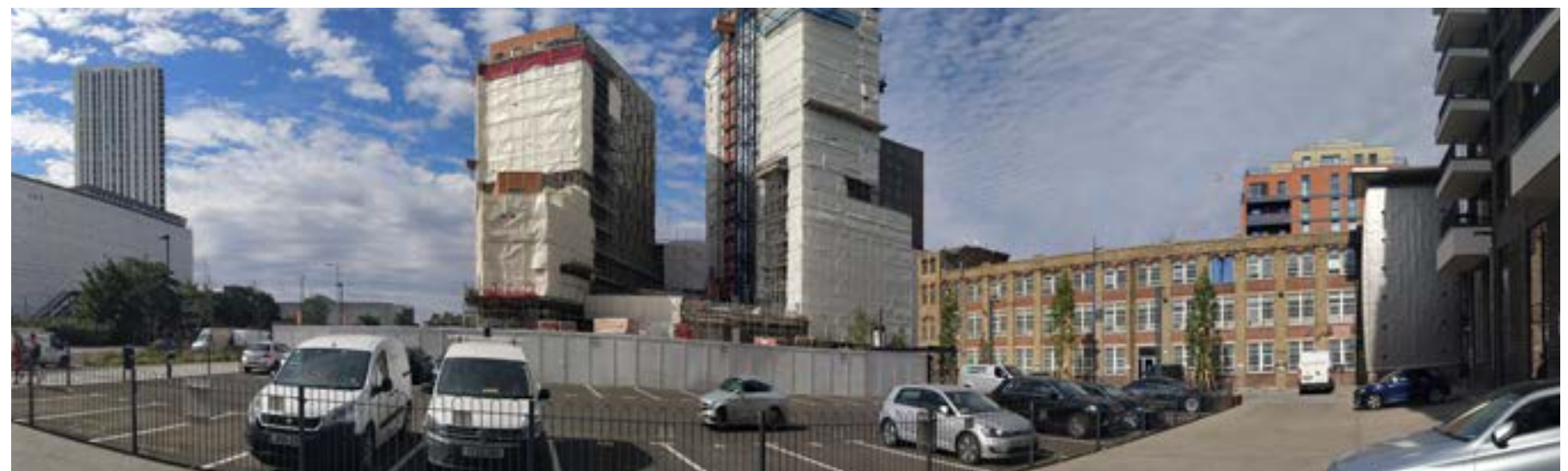
Panoramic photo of site today with Berol House and the existing and emerging neighbouring context.
