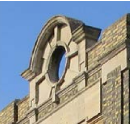
BEIGE CONCRETE DETAILS
