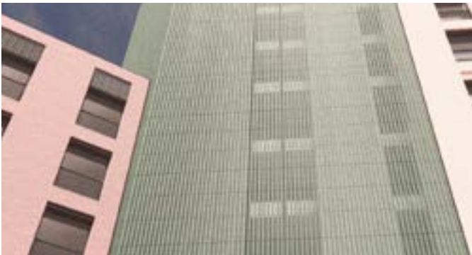
The exposed core allows daylight to the corridors and views out
