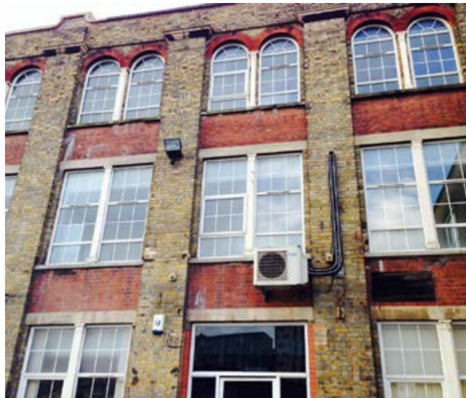
View of the rear elevation
