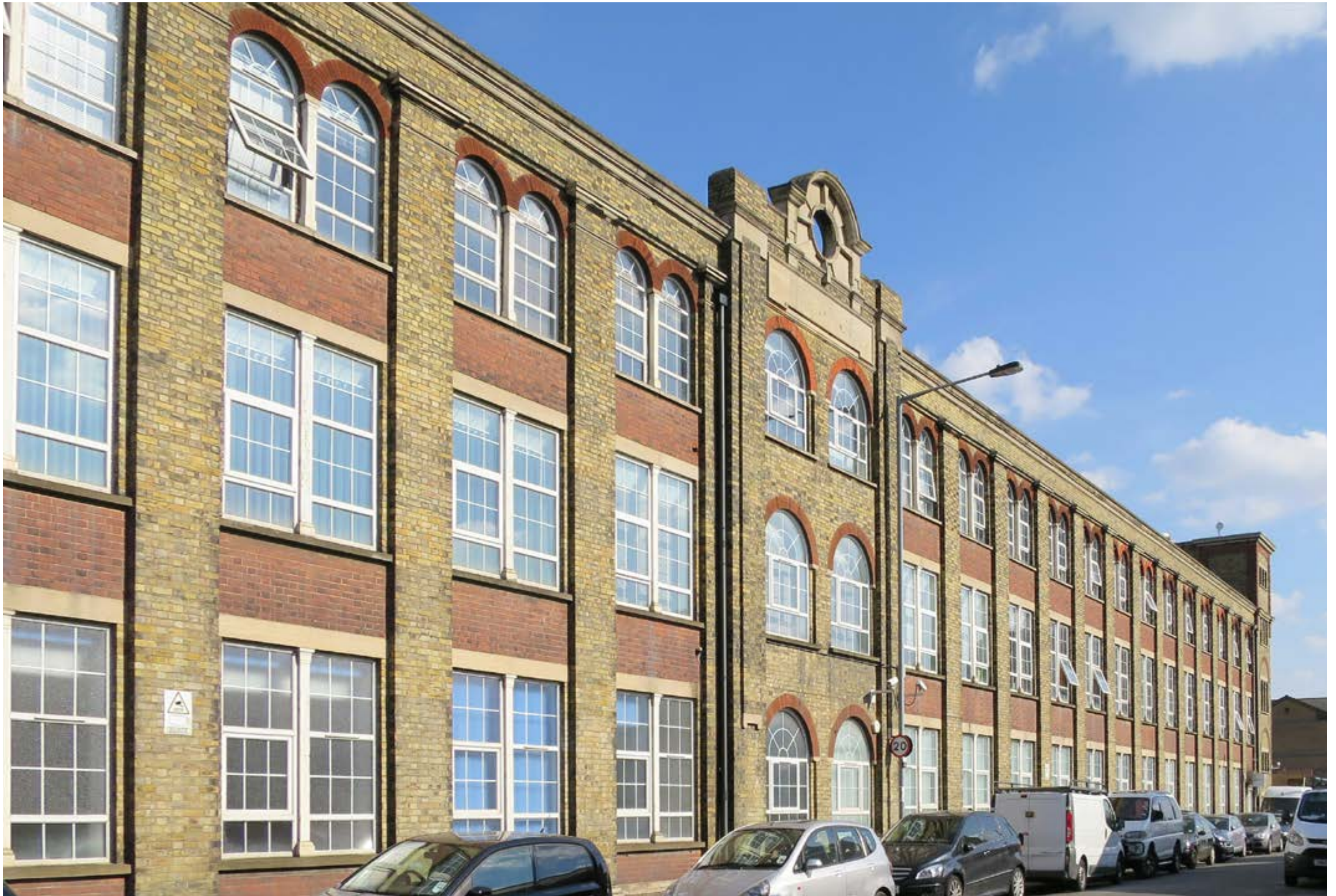
Photograph of the existing building
