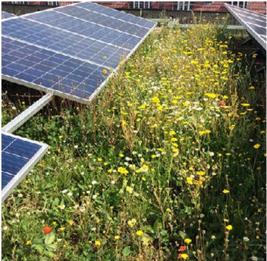
2 — Example of a biosolar roof
