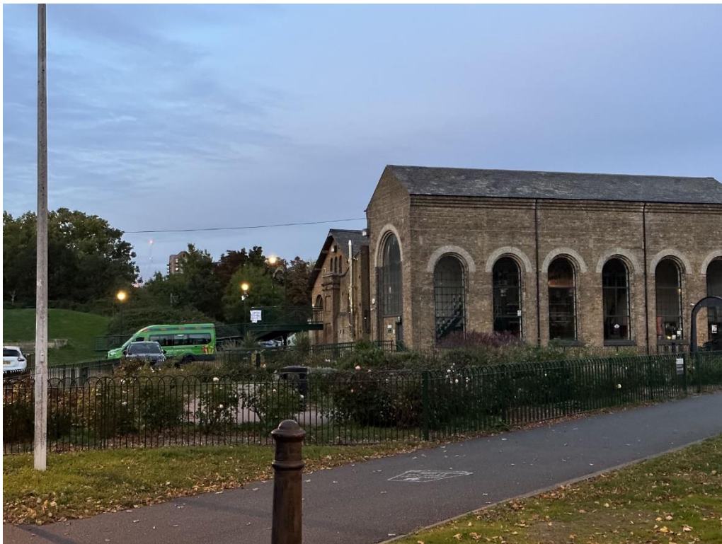
Figure 5.8 Pumping Station Building and Engine looking north towards the site
