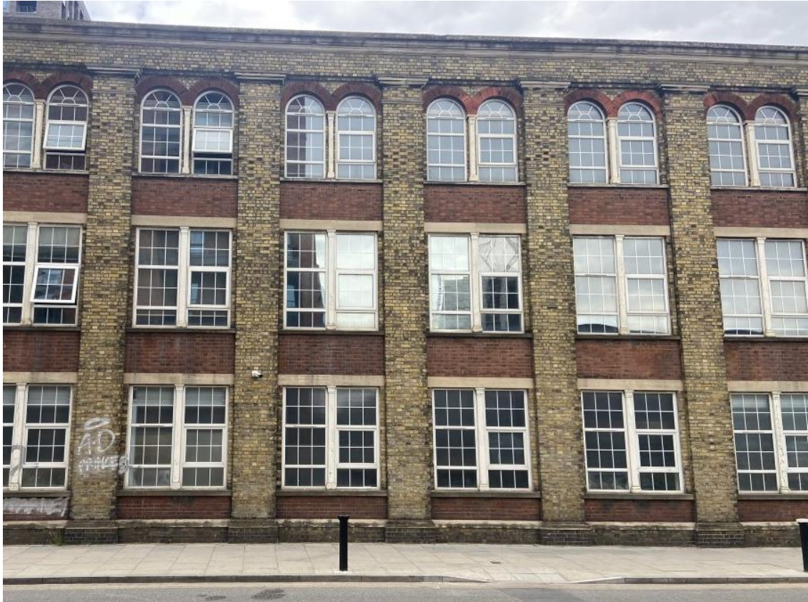
Figure 5.2 Elevational detail to Berol House showing pilaster and fenestration pattern
