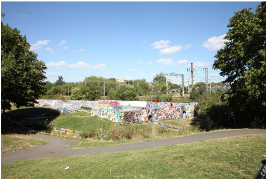
Figure 5.9 Setting of the Pumping House, looking south from the building
