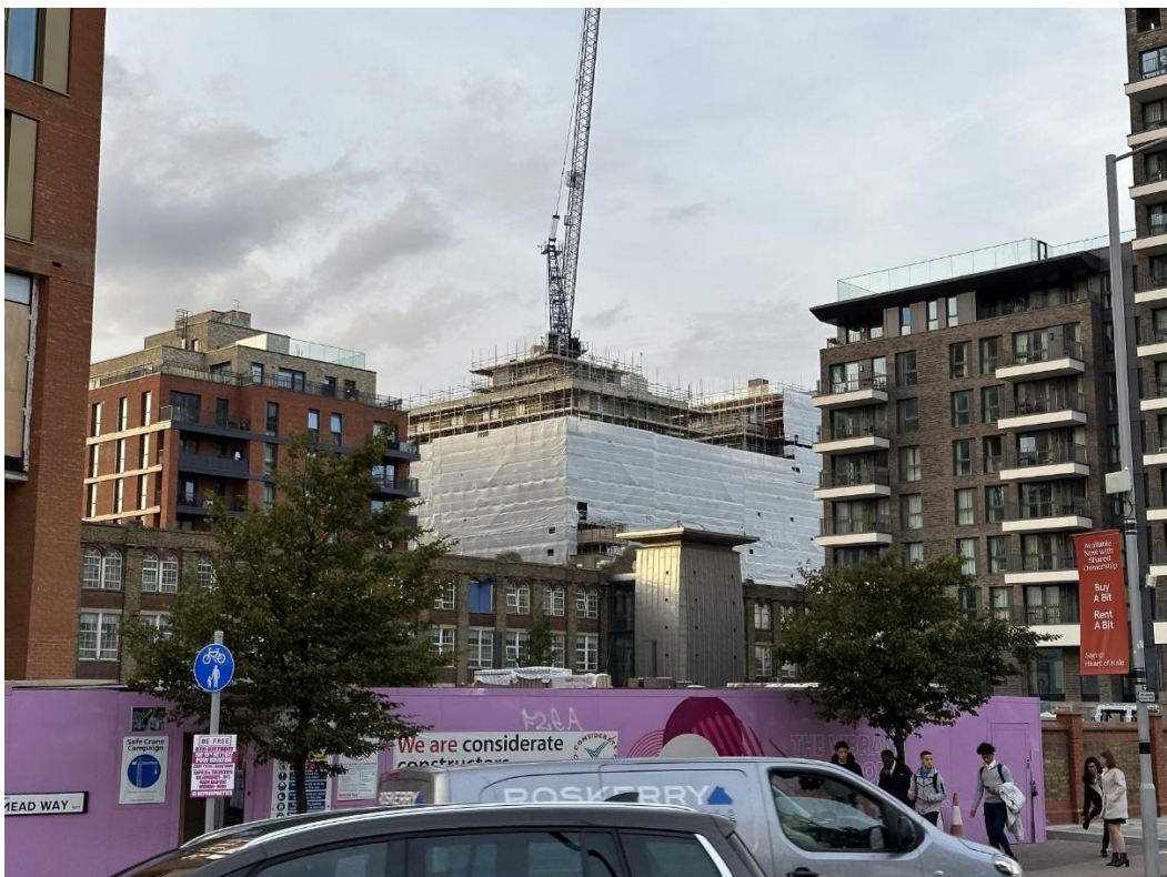
Figure 4.3 Looking west across the site for 2 Berol Yard in the foreground with Berol House in the background. This image again shows the much-changed setting of Berol House which is now surrounded by taller development and the vacant 2 Berol Yard site
