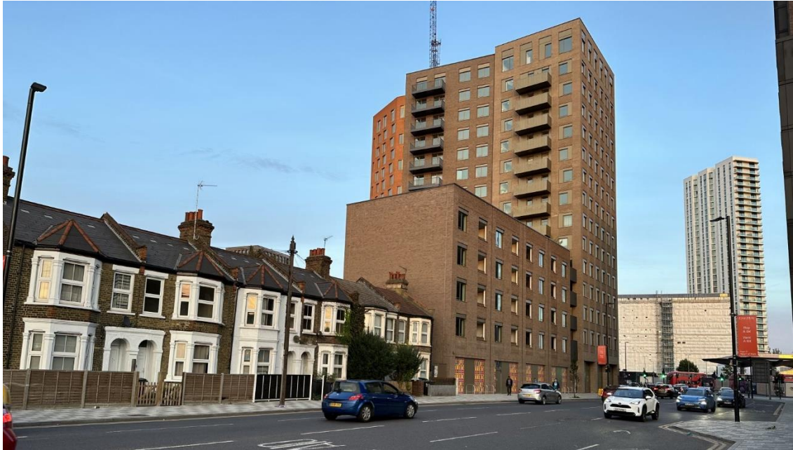
Figure 5.7 Terraced houses to the left, seen looking towards the site from the south-west. The changing context is readily visible in the mid and background
