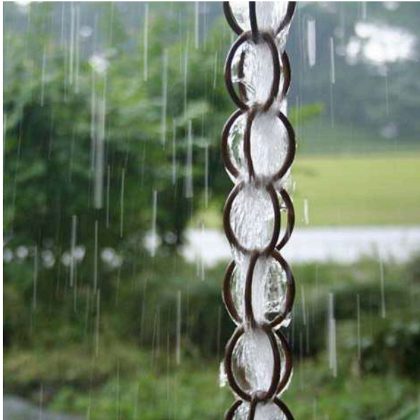
Rainwater running down a chain drain
