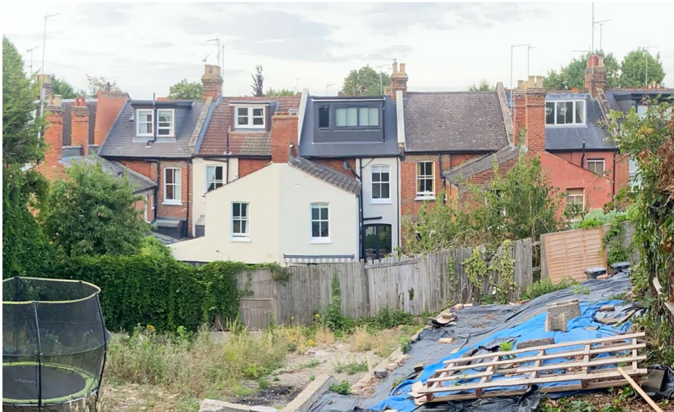
8. VIEW TOWARDS THE BOUNDARY WITH TIVOLI ROAD HOUSES.
