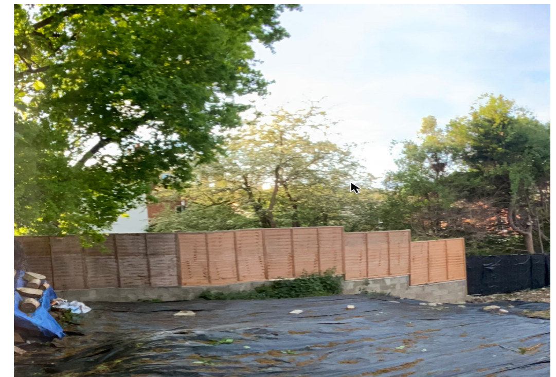
20. VIEW NORTH TOWARDS GLASSLYN ROAD FROM SEMI-DETACHED MASTER BEDROOM
