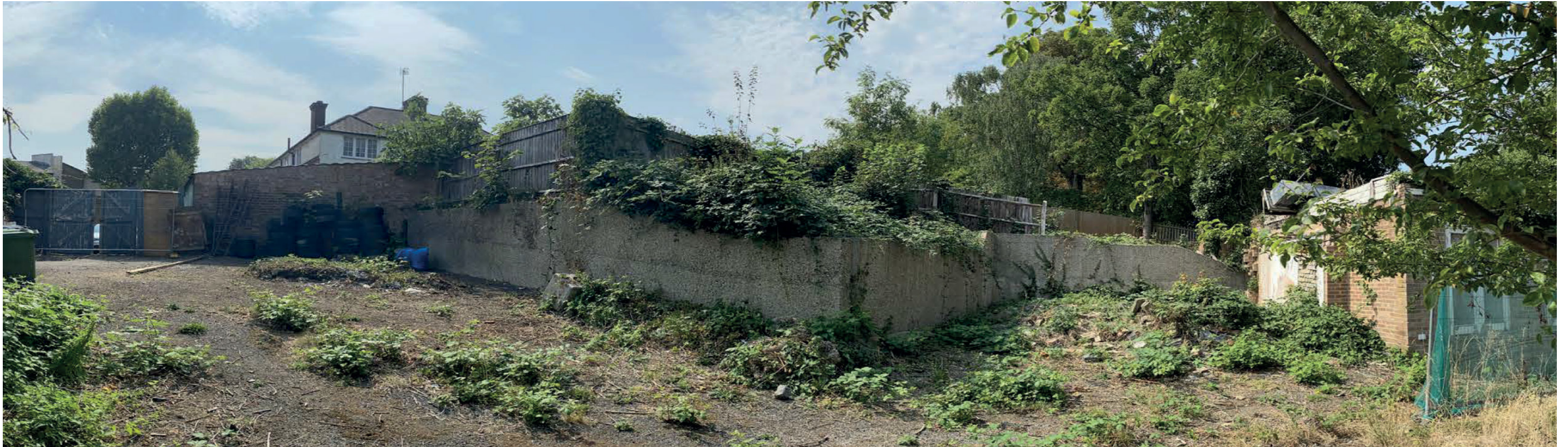
6. VIEW OF RETAINING WALL & FENCE TO REAR GARDEN OF 60 WOLSELEY RD
