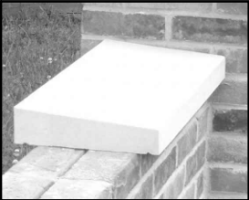
Item 3, natural finish concrete coping stones to cap parapet wall
