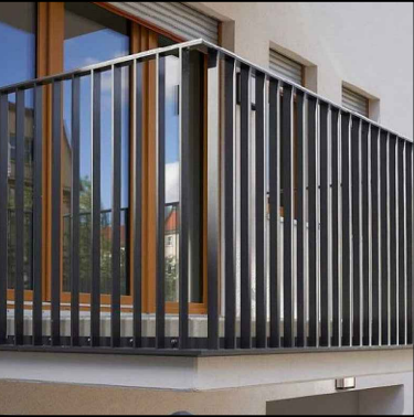
Item 9, black colour metal railings
