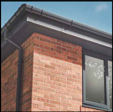
Item 4, dark grey colour fascia and soffit board, with grey gutter and downpipes including soil pipes
