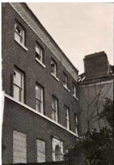
Figures 18 and 19 showing Front and Rear Elevations. All windows were broken and the photographs show the ground floor openings blocked up for safety.
