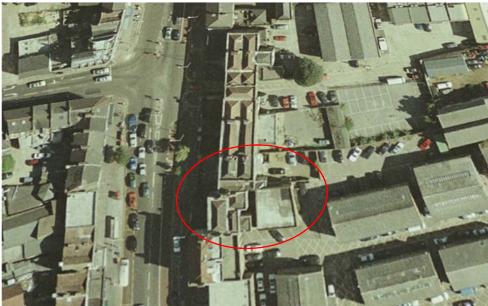
Figure 32 – 1999 Google Aerial Photograph showing the Industrial Estate and rear extension to Number 792.
