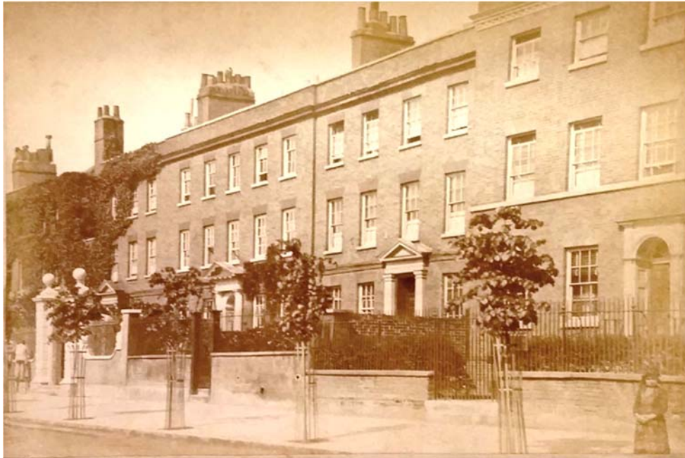
Figure 12 - 1880-1885 Photograph of frontages of Nos. 792-800 High Road. Note that No.794 and 798 have matching aedicules (symmetrical each side of Percy House). The windows are all 6-over-6 vertical sash windows, prior to the change to single plate glass panes in the 1890s.
