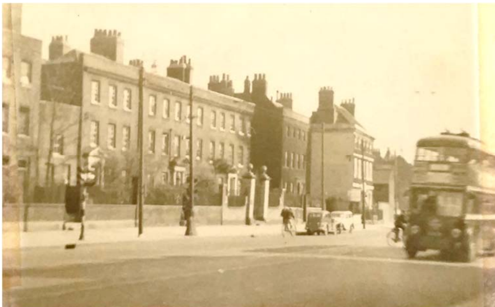
Figure 13 - May 1939 of 790-800 High Road. Number 792 projects forward, covered in ivy. Nos. 794 and 798 are symmetrical, each side of Percy House
