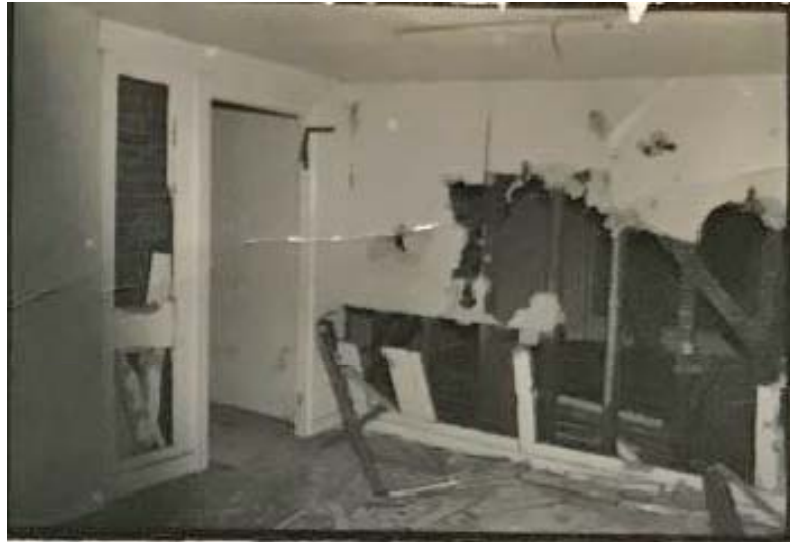
Figure 29 (Right) Showing extensive plasterboard surfaces on the second floor.
