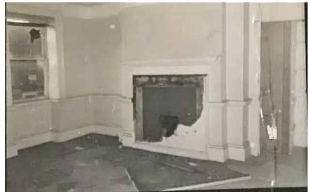
First Floor Firesurround. Comparison with 1977 photograph (right) shows modern infill of no significance of former doorway between No. 792 and 794.
