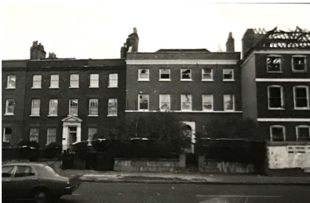
Figure 17 – Numbers 790 to 794 after the fire.
