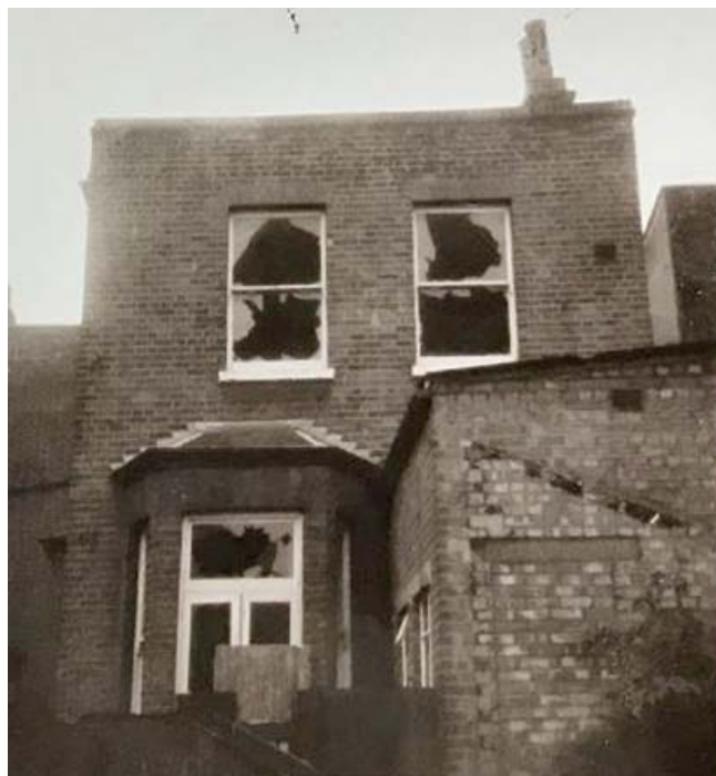
Figures 18 and 19 showing Front and Rear Elevations. All windows were broken and the photographs show the ground floor openings blocked up for safety.
