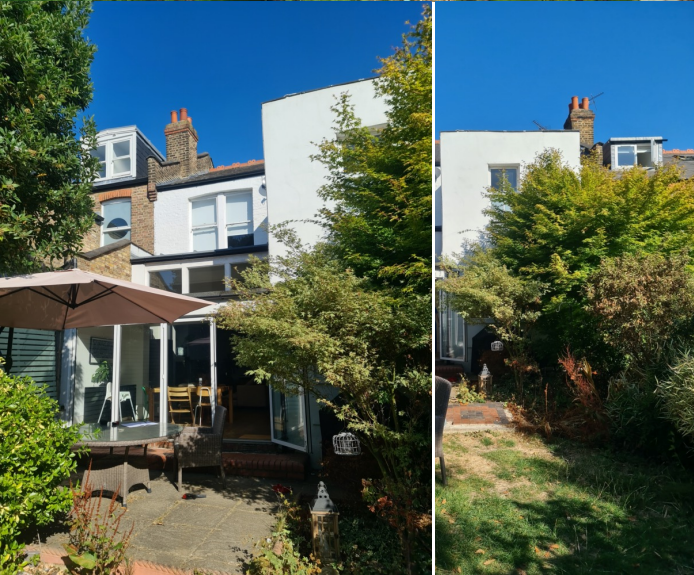
Existing Rear Elevation to 86 Muswell Road, N10 2BE
