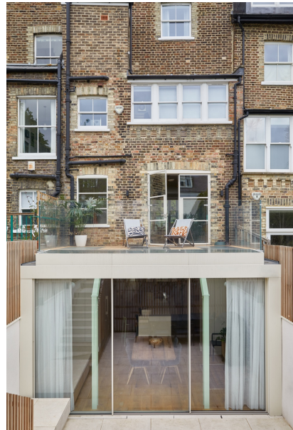
Work Sample 2 Christchurch House – Stone clad rear extension, North London
