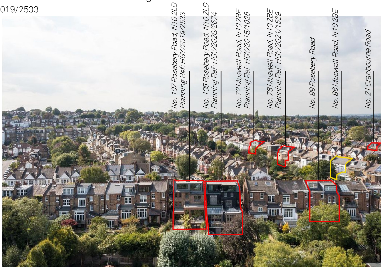
Drone view of No. 86 Muswell Road surrounded by at least 6 identified properties along adjacent streets with enlarged rear dormers.
