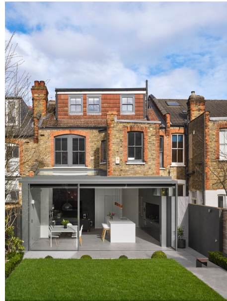
Work Sample 4 Dukes House – Rear extension, North London
