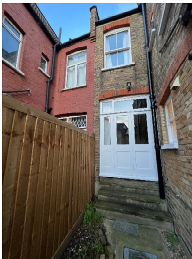
The closeness of the bedroom window 143 Muswell Ave to the proposed building site
