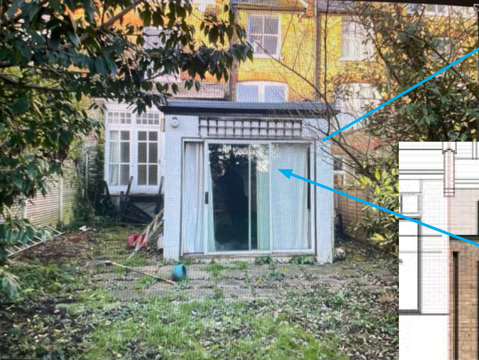
Current View towards property
