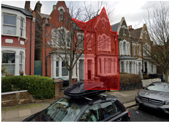
View from Cavendish road
