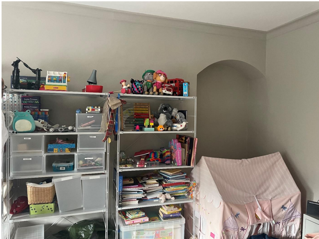
6.0 Internal ground floor. Flues in existing wall serving fireplaces?
