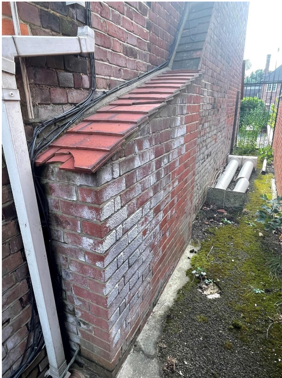
4.0 Newer rear Chimney breast extension.
