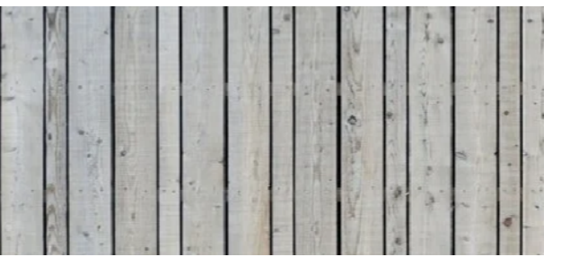
150mm x 19mm Board-onboard vertical timber (Larch) cladding to north and east elevations of the pavilion
