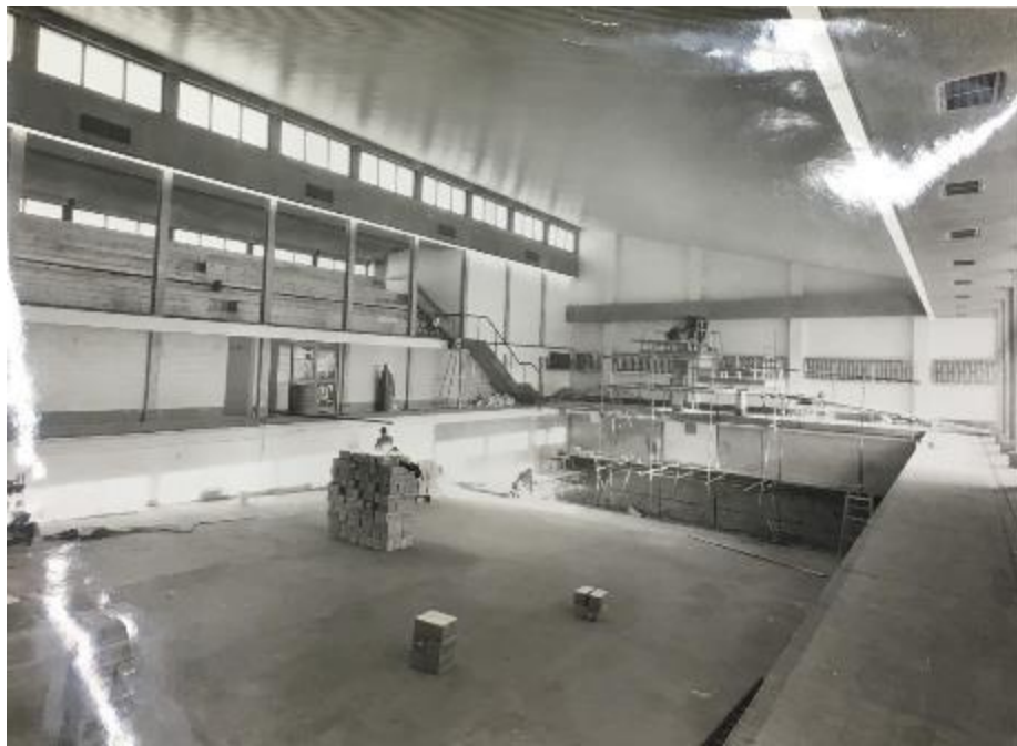
Figure 11. Mallinson Swimming Pool Under Construction.
