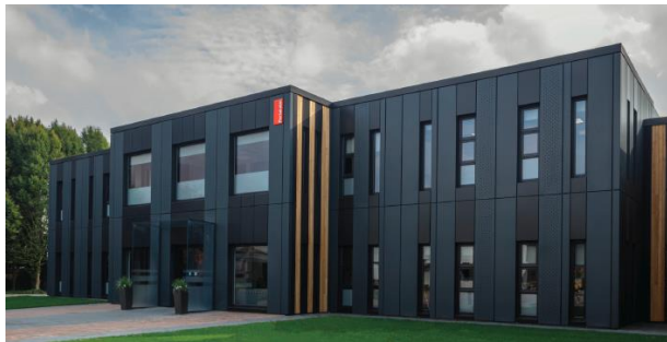
Figure 13 Modular building with external insulation and cladding.
