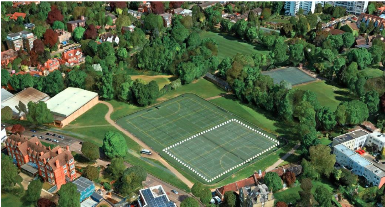
Figure 4 Aerial view of synthetic pitch area.
