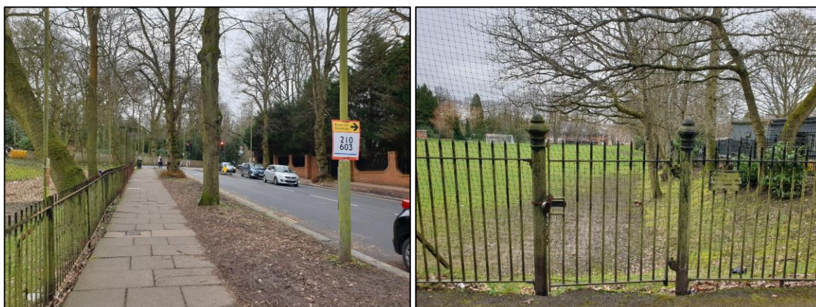
Figure 2.5 Footway on Hampstead Lane and pedestrian gate
