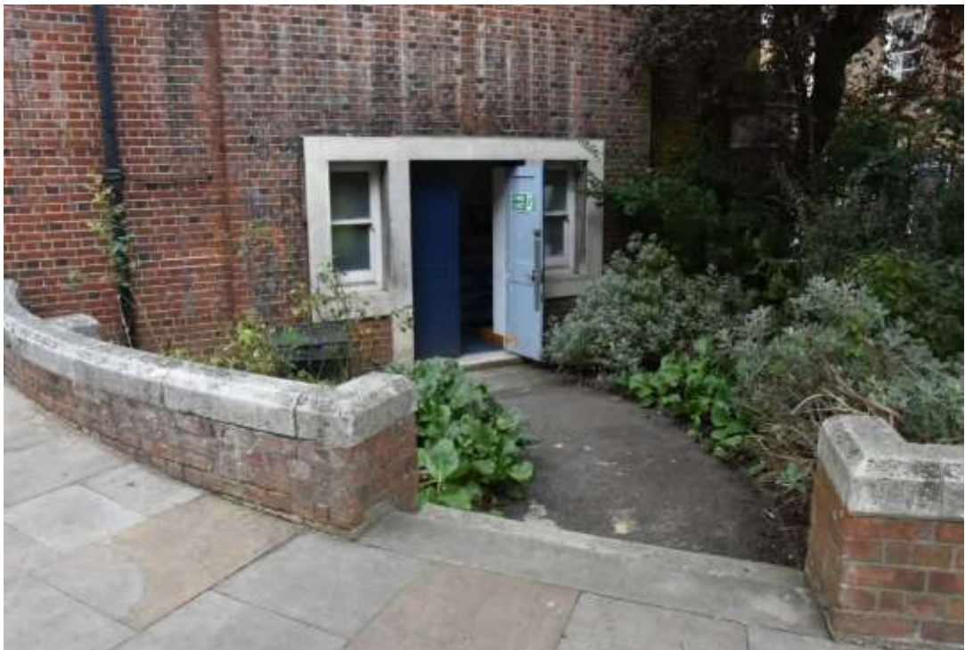
Fig.45: Access to the lower level of the Science Building. Facing NE
