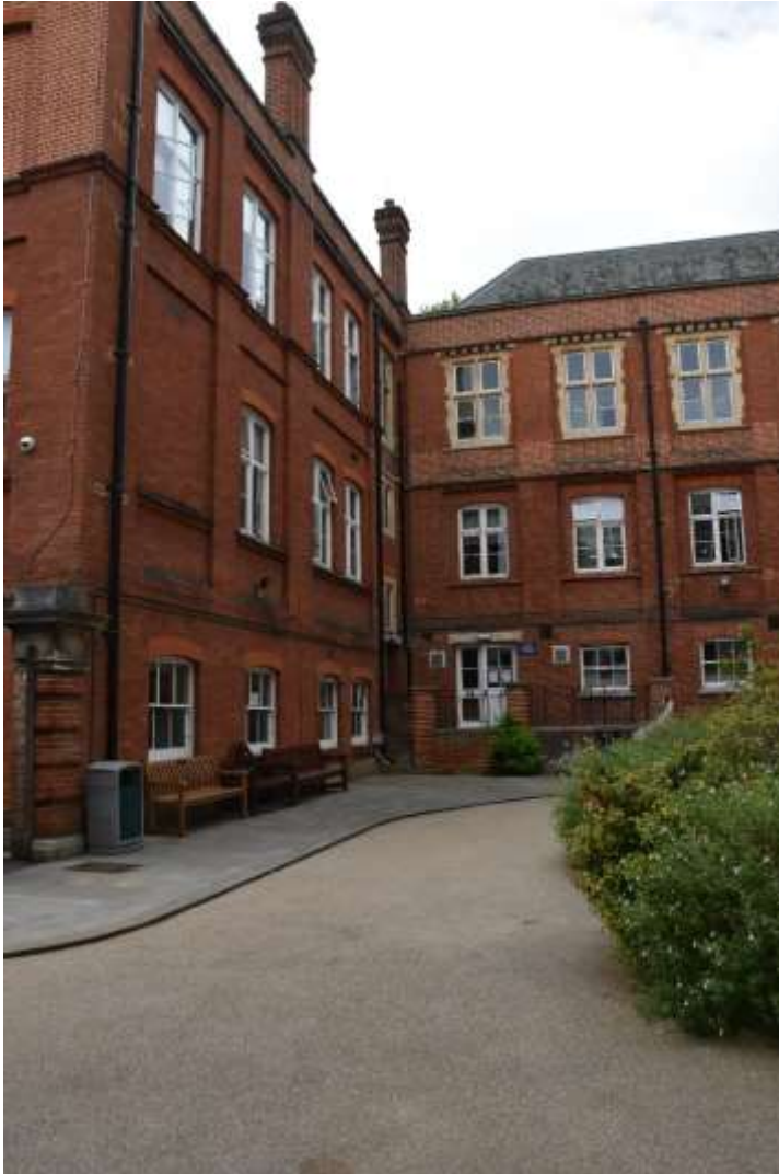
Fig.43: Central Hall and the Link Block. Taken from the Science Quad facing W
