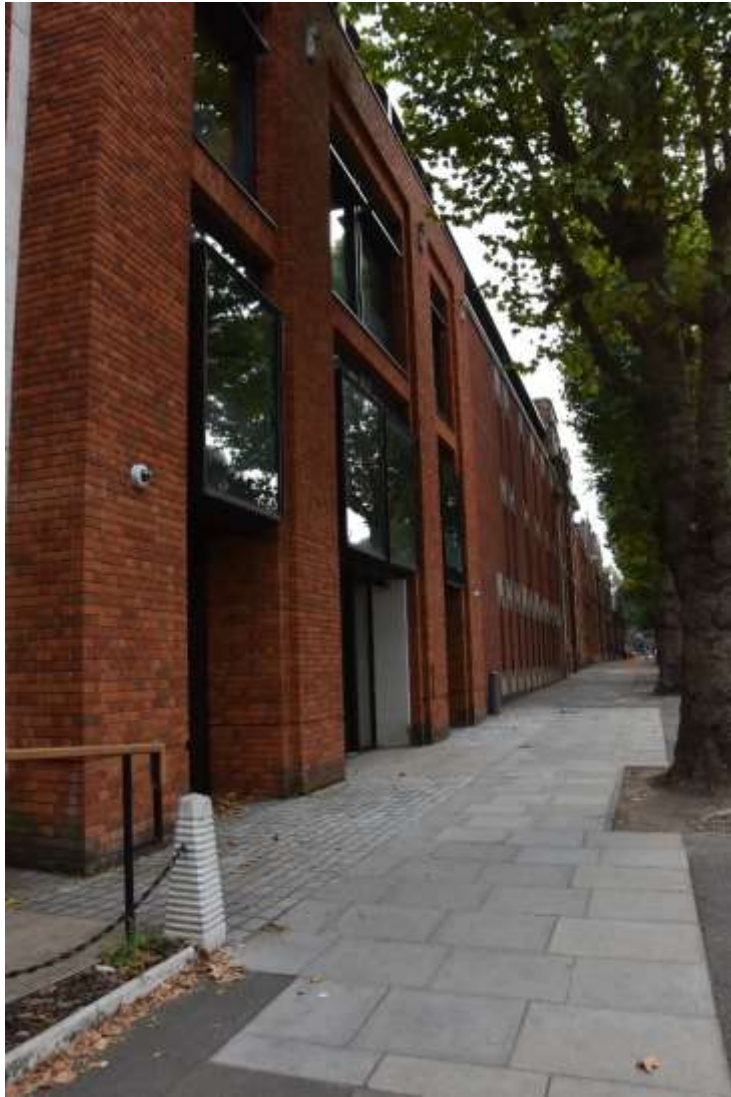
Fig. 37: View of the Charter Building, looking towards the Garner Building. Facing S
