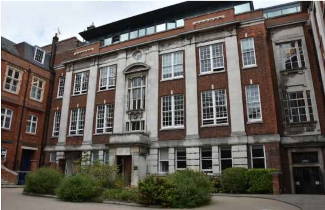
Fig.44: Science Building. Facing approximately NNW
