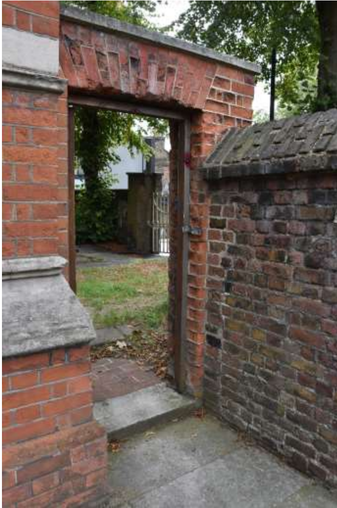
Fig.53: Gateway on the western side of the Chapel leading to the burial ground. Facing SSW
