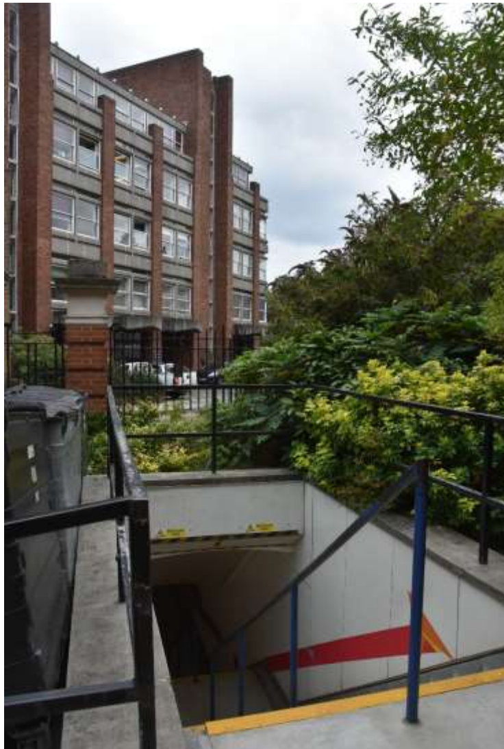
Fig.46: Tunnel linking the Island Site to Dyne House. Facing ESE
