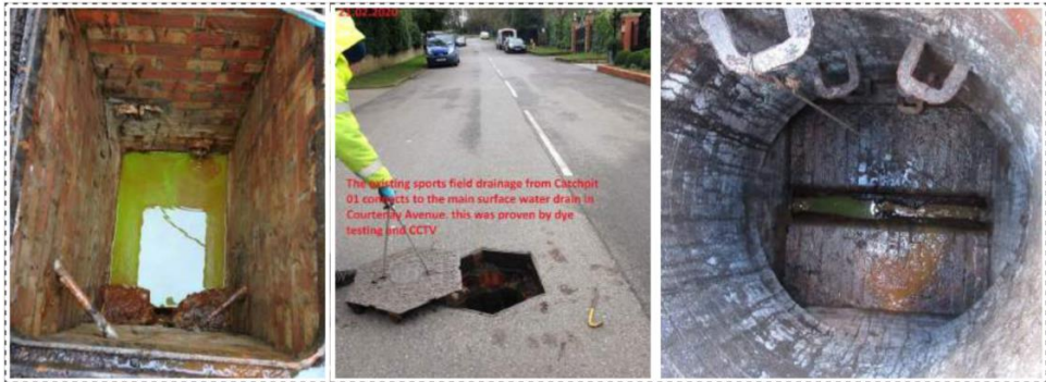
Figure 7 – Existing Drainage Located – Left Catchpit 1 on site. Middle & Right Courtenay Avenue
