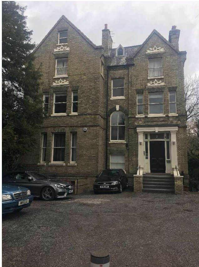
Figure 37. 2 Bishopswood Road to the south of the site.
