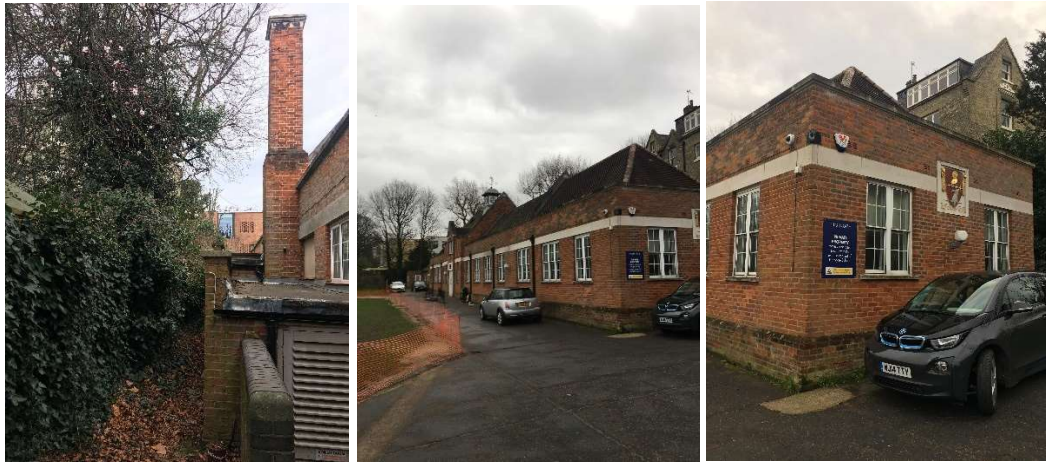
Figure 27. Exterior facades of the site. Note stone banding with rebuilt brick above to the parapet. Relocated plaque to the western end of the building. Small brick ancillary structures to the rear containing servicing altered during the 1990s.
