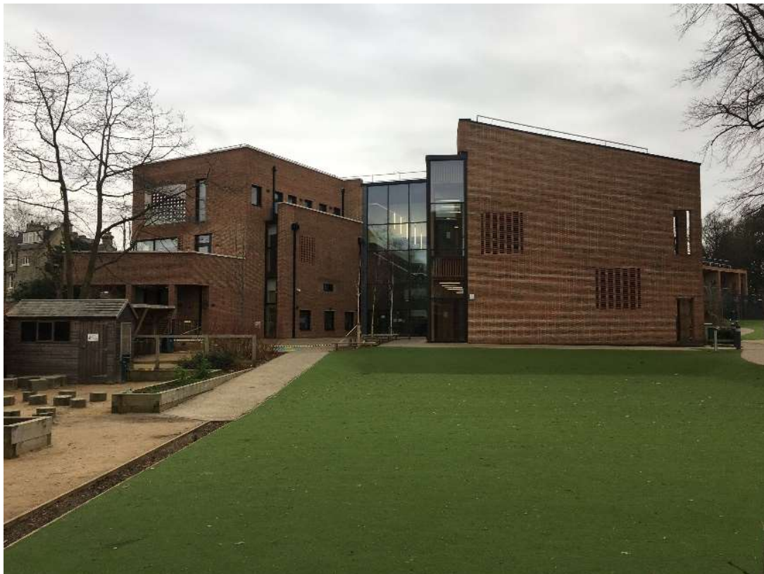
Figure 35. New junior school buildings to the west of the site. Note bold massing and use of glazing to create voids and variety within the form.
