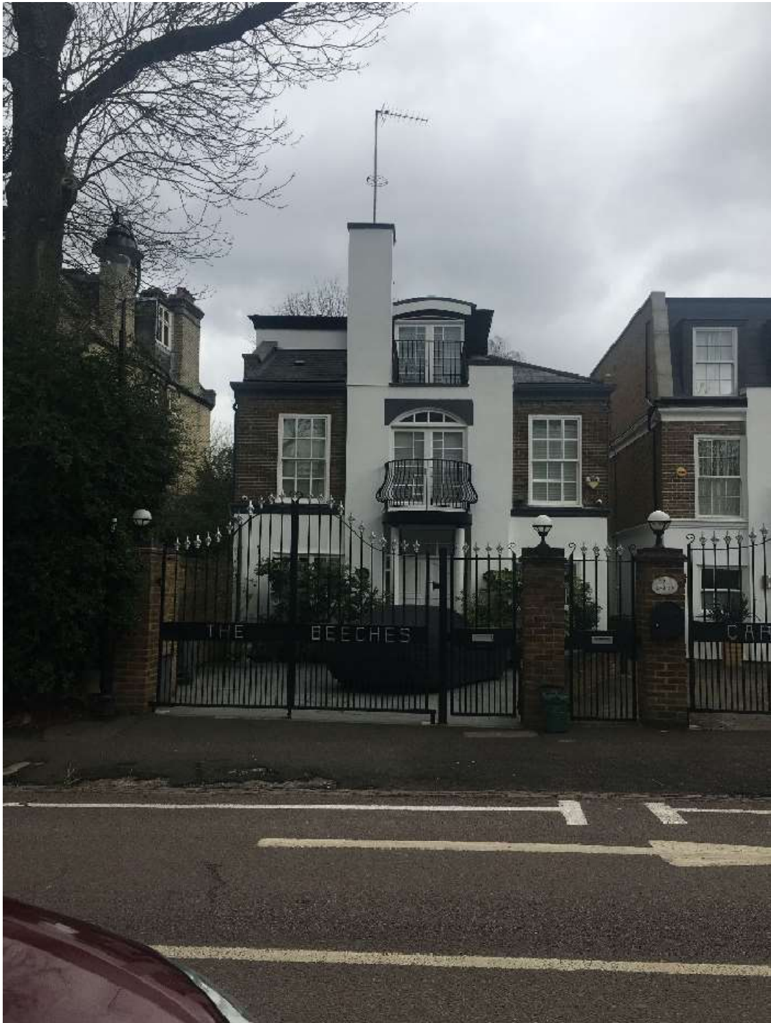
Figure 36. View of the 1980s the Beeches Villa, creating a contemporary but contextual aesthetic to Bishopswood Road to the south of the site.
