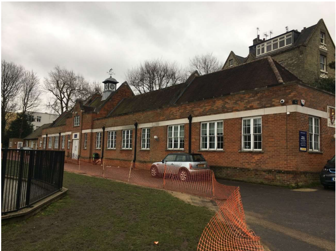
Figure 26. RMC main façade seen from the North. Note red brick exterior, with central timber cupola and raised parapet to the central bays. Stone banding can be seen below rebuilt brick parapet. Note western extension includes rebuilt roof above, with original gable end visible to roof line. To the east the later single storey extension can be seen. Fenestration comprises late twentieth century replacement timber sashes.
