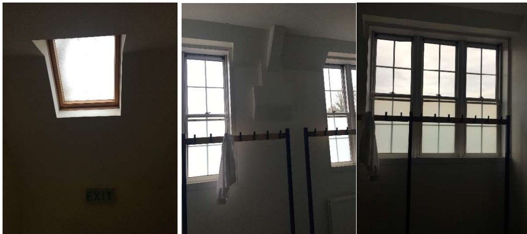
Figure 29. Interior views of the RMC showing fenestration, including skylights and timber sashes, all dating the late twentieth century refurbishment.
