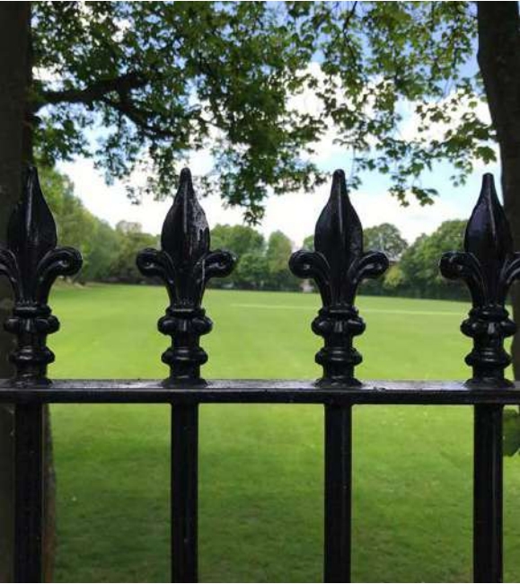
Fig. 39: Existing replacement railings to the Eastern boundary of Far Field, along Courtenay Avenue.
