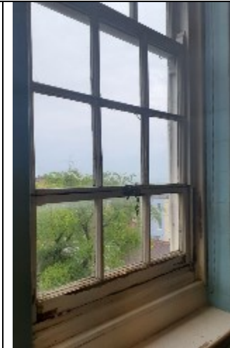
Image 7 Timber Window Frame
