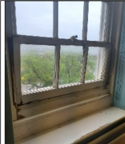
Image 6 Timber Window Frame
