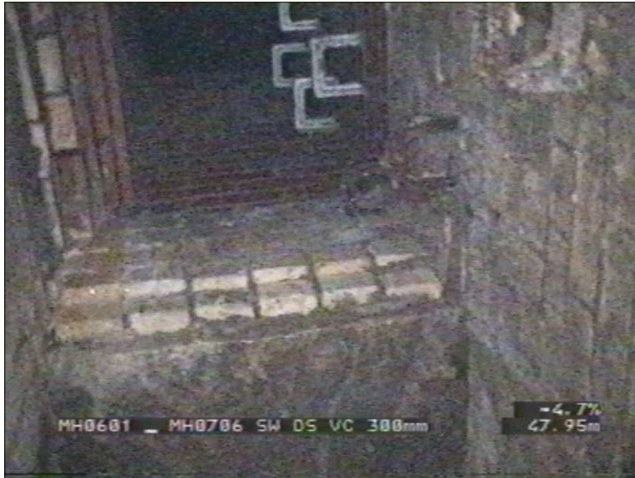
Photo: 50_7a, Tape No.: 002, 23:48:01 47.73m, Finish node type, manhole, reference number: 0706
