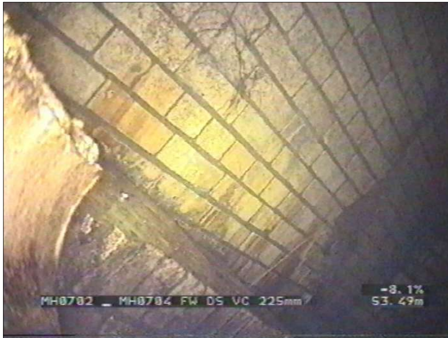
Photo: 61_6a, Tape No.: 002, 23:56:06 53.49m, Finish node type, manhole, reference number: 0704
