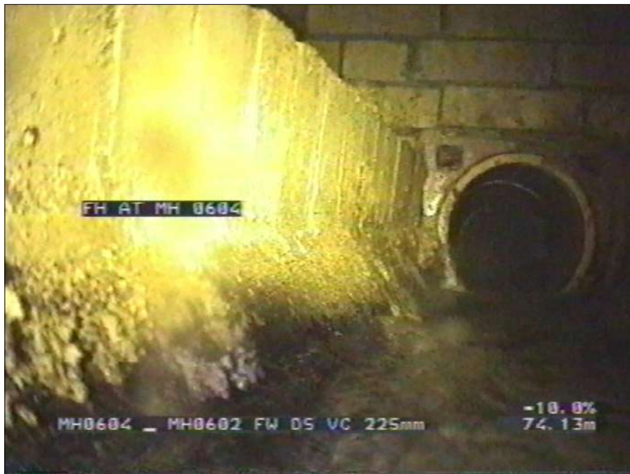
Photo: 7_7a, Tape No.: 002, 23:30:15 74.13m, Finish node type, manhole, reference number: 0602
