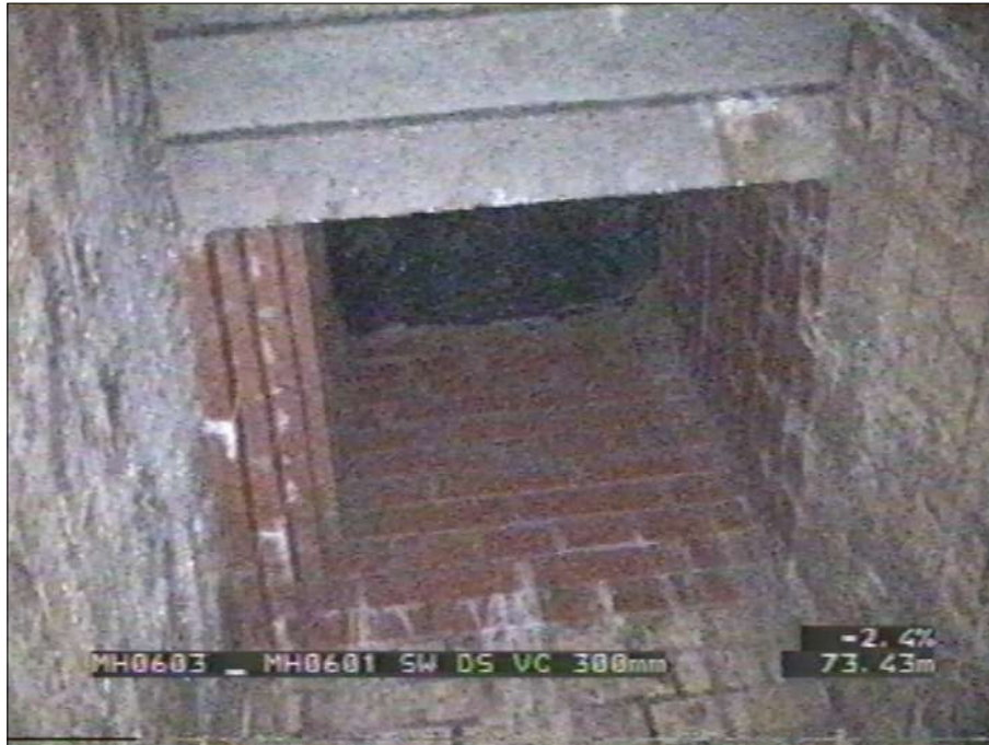
Photo: 43_26a, Tape No.: 002, 23:43:43 73.43m, Finish node type, manhole, reference number: 0601
