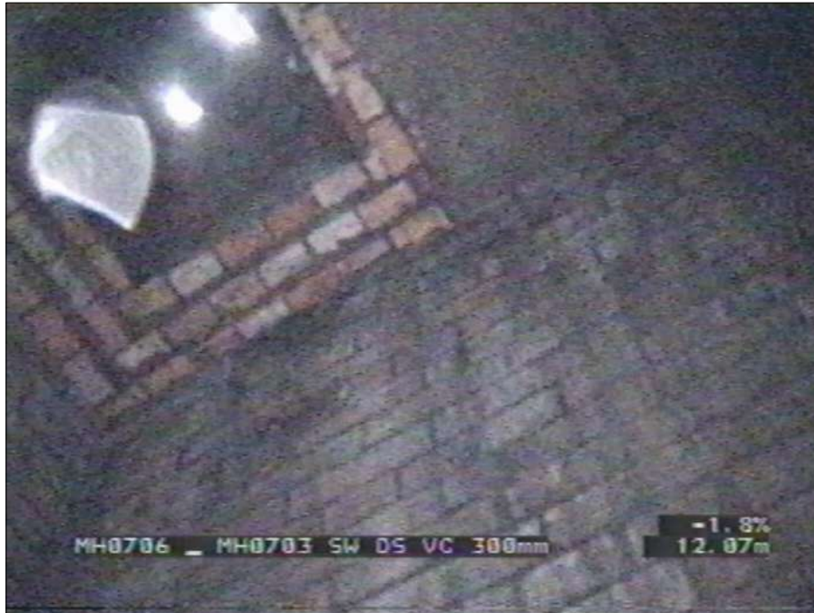
Photo: 55_5a, Tape No.: 002, 23:50:11 12.07m, Finish node type, manhole, reference number: 0703
