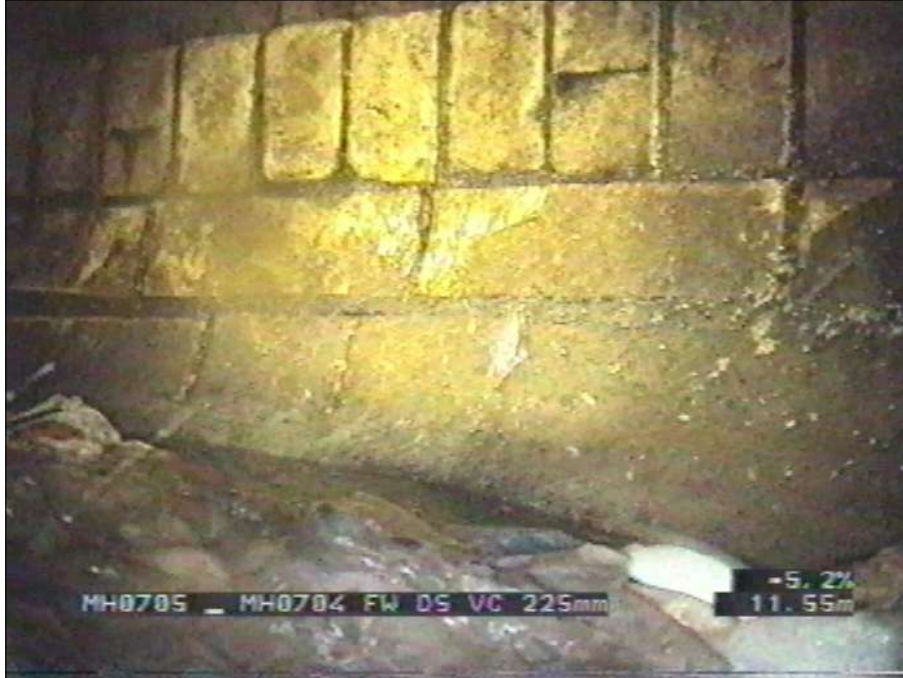
Photo: 17_5b, Tape No.: 002, 23:38:14 11.55m, Finish node type, manhole, reference number: 0704
