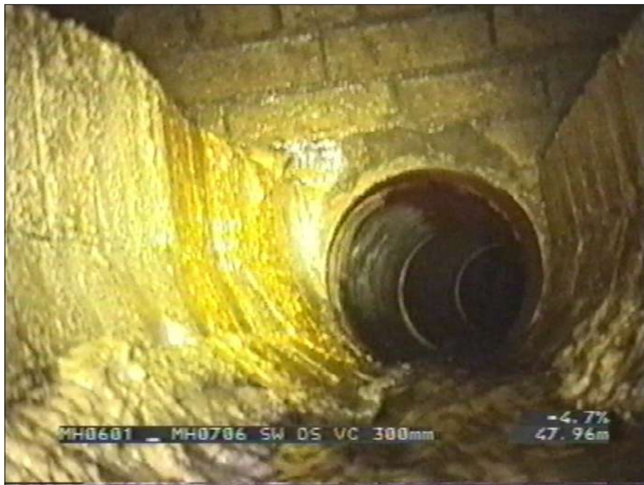
Photo: 50_7b, Tape No.: 002, 23:48:01 47.73m, Finish node type, manhole, reference number: 0706
