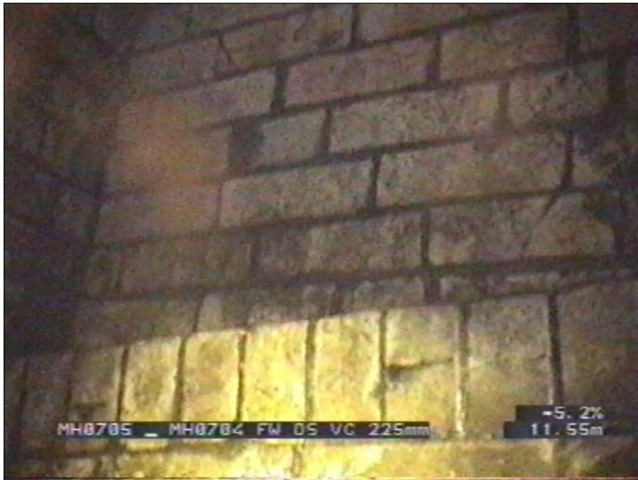
Photo: 17_5a, Tape No.: 002, 23:38:14 11.55m, Finish node type, manhole, reference number: 0704
