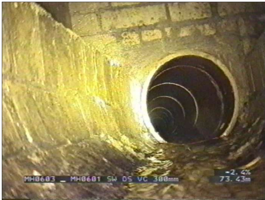
Photo: 43_26b, Tape No.: 002, 23:43:43 73.43m, Finish node type, manhole, reference number: 0601
