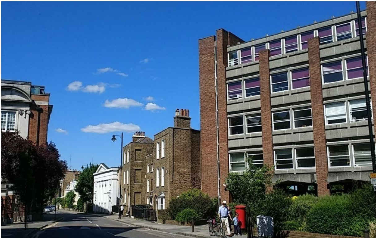
View on Southwood Lane looking north, Science East Wing on the left, Dyne House on the right
