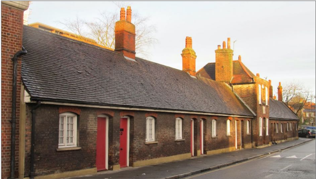
View on Southwood Lane of the almshouses
