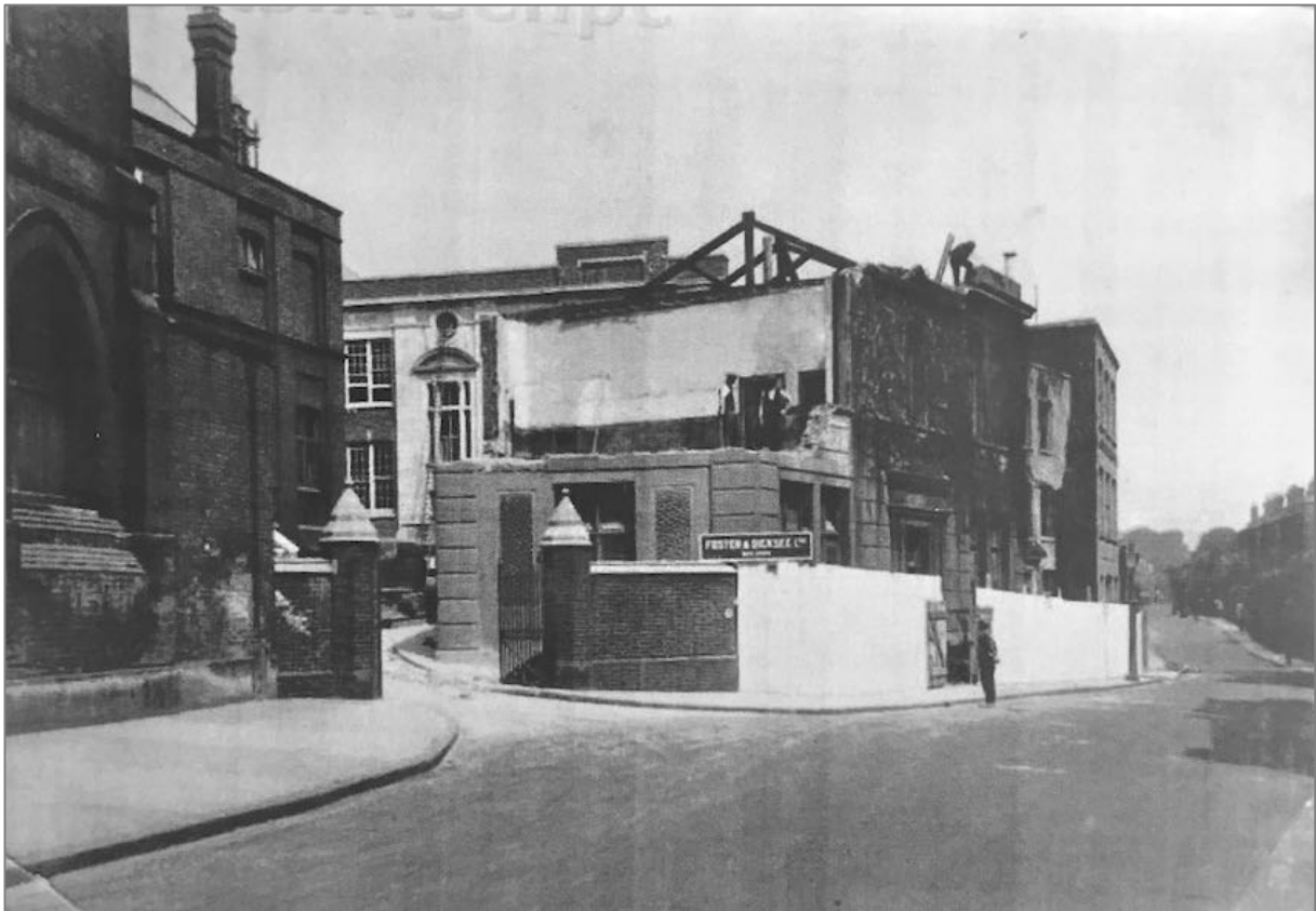
Photograph taken circa 1928, with demolitions in progress for East Wing site
