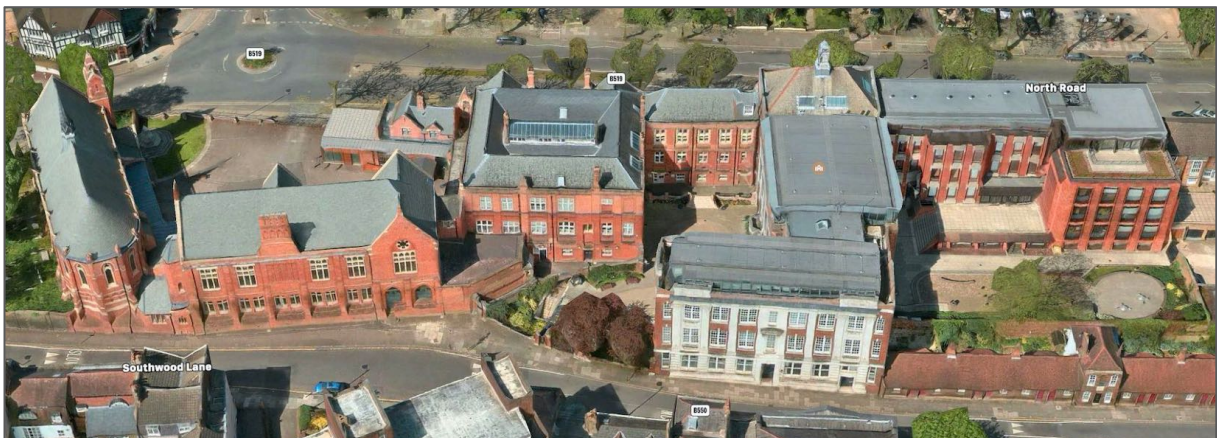
Aerial view of the whole campus from the east
