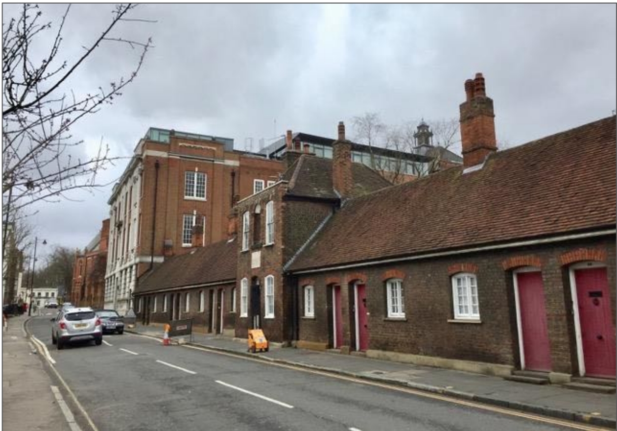
Street view on Southwood Lane of the Science Buildings from the north
