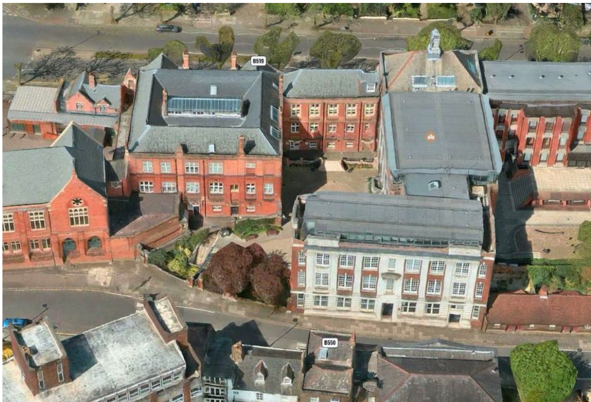
Aerial bird's eye view of the Science Buildings from the east, on Southwood Lane
