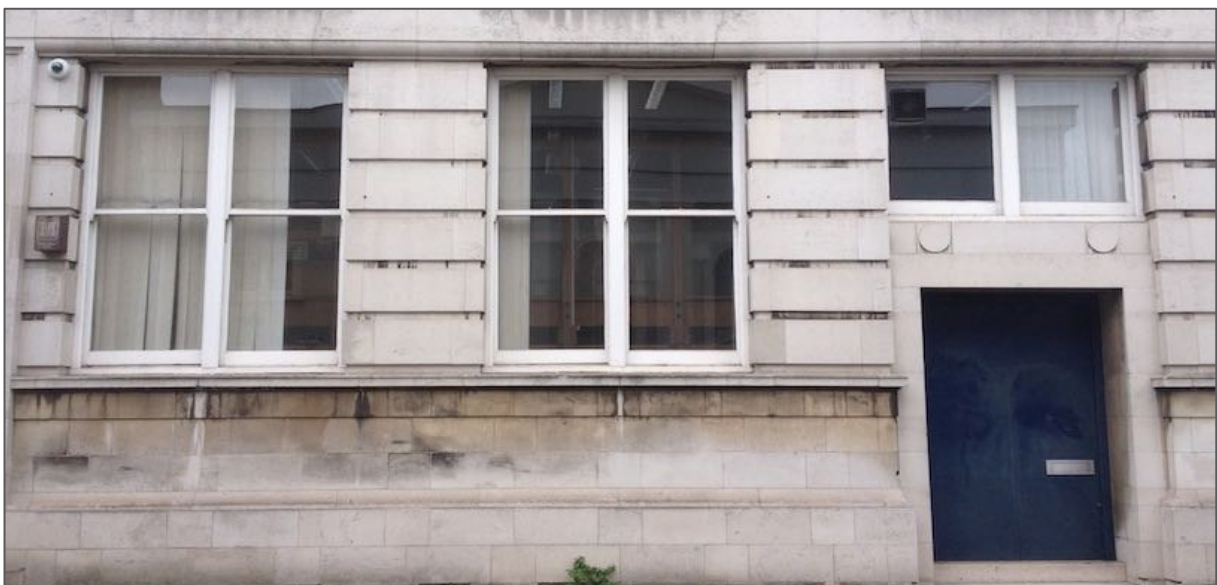
Detail view of the east elevation of East Wing from Southwood Lane
