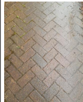
Image 5 External Brick Pavement
