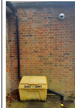
Image 4 External Brick Wall
