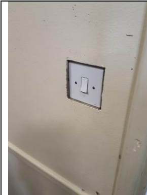
Image 17 Plasterboard Internal Walls
