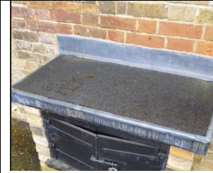
Image 25 Bituminous Material
